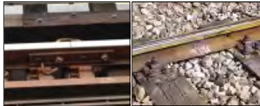
Jointed versus Welded Rail
