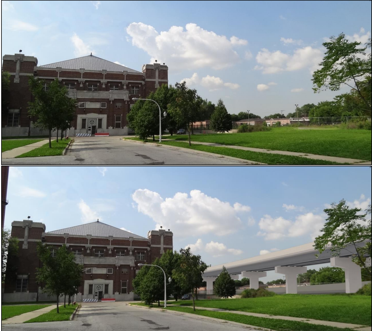
Figure 4-25: Photo of Existing Conditions and Photo Simulation of the Union Pacific Railroad Alternative East Option Elevated Track Structure adjacent to the Roseland Pumping Station, Facing South on Harvard Avenue
