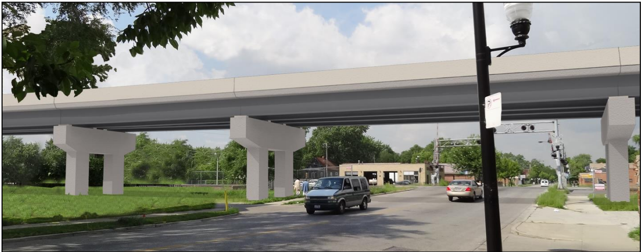
Figure 2-3: Photo Simulation of Union Pacific Railroad Alternative East Option at 111th Street Facing West - Typical Proposed Elevated Structure
