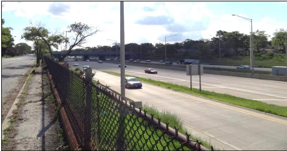
Figure 4-11: Photo Facing East, North of I-57 near 98th Street and Lowe Avenue
