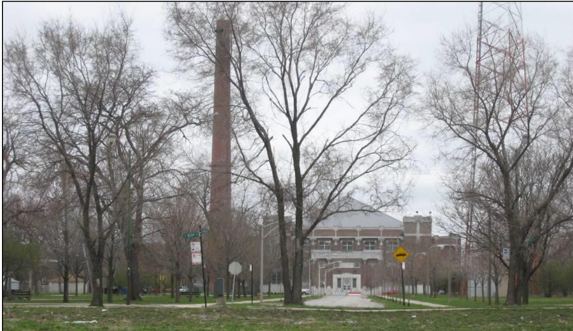
Figure 8-7: Photo of Block Park with the Roseland Pumping Station in the Background (Facing South)
