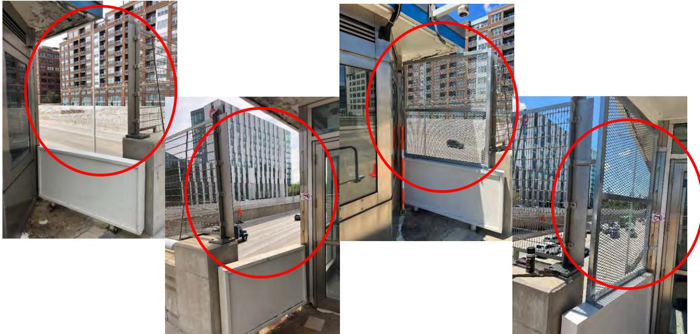
**UIC/Halsted- Install high barrier fencing on existing railing for safety.**
