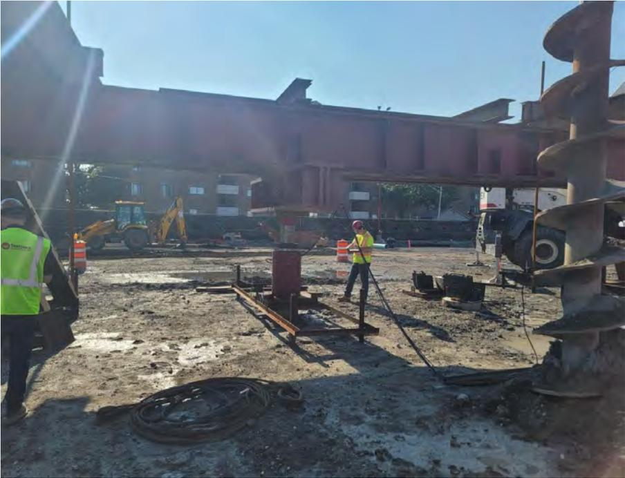
**Pile Pressure Testing Setup**
