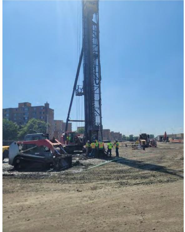
**Pile Drilling Rig**
