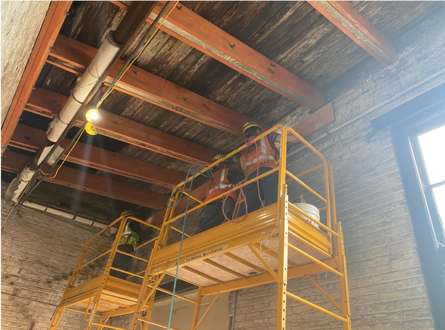
**Roof Joist Additional Support Installation**
