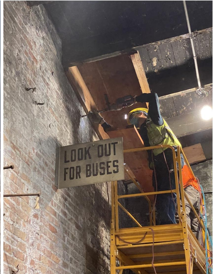
**Roof Joist Additional Support Installation**
