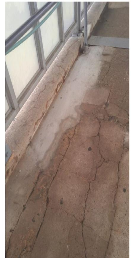
**Western (Blue Line Congress) Repair Areas of Loose & Spalling Concrete of the Ramp**
