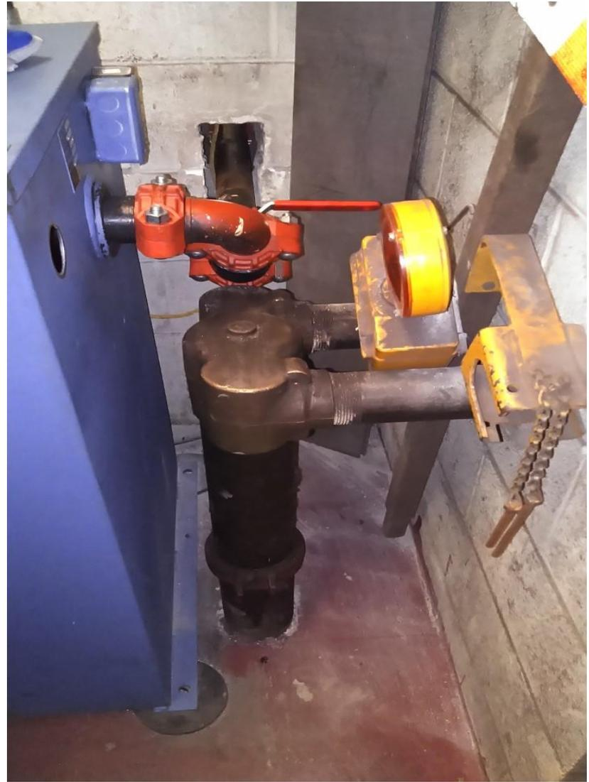
**Elevator #1 - New hydraulic pump with new lines to the elevator pit**
