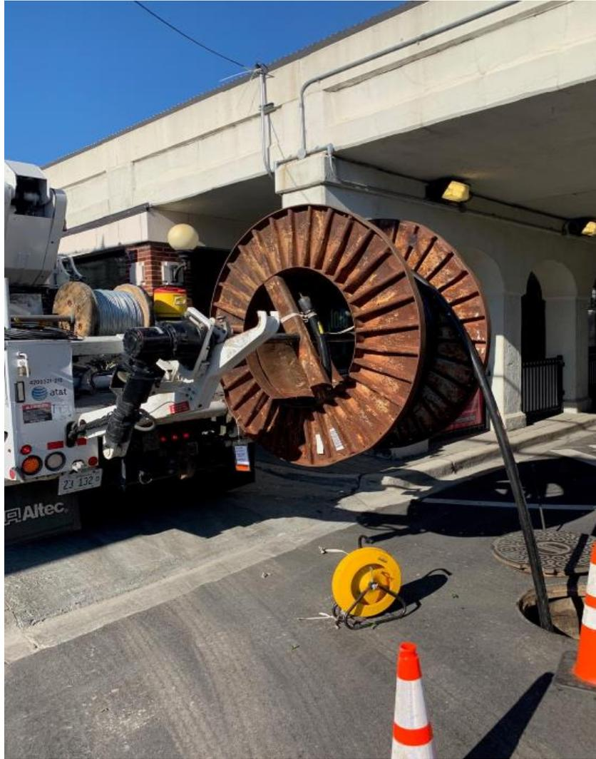
**AT&T Pulling Copper at Argyle Manhole**
