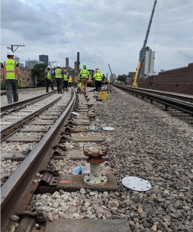
Thorndale interlocking work, installation of contact rail chairs,
