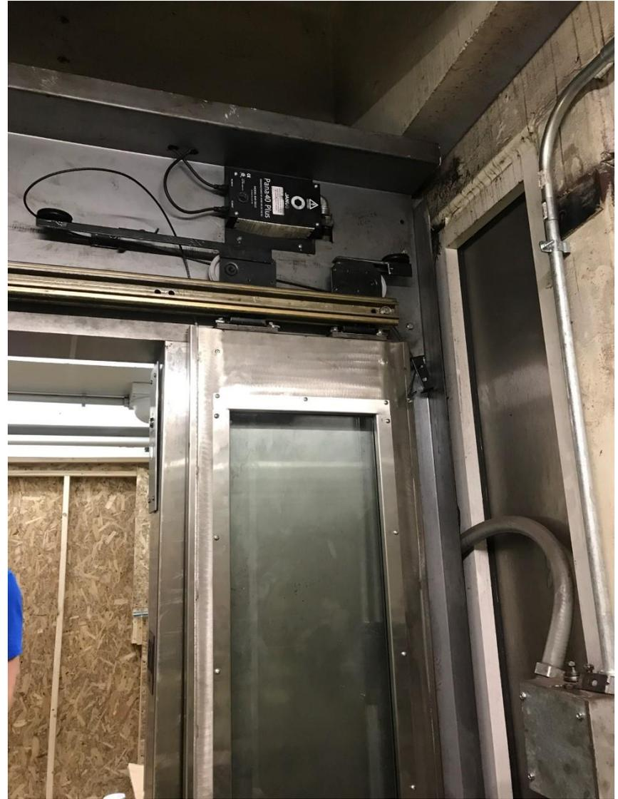
**Elevator #1 - New elevator doors and hardware installation**
