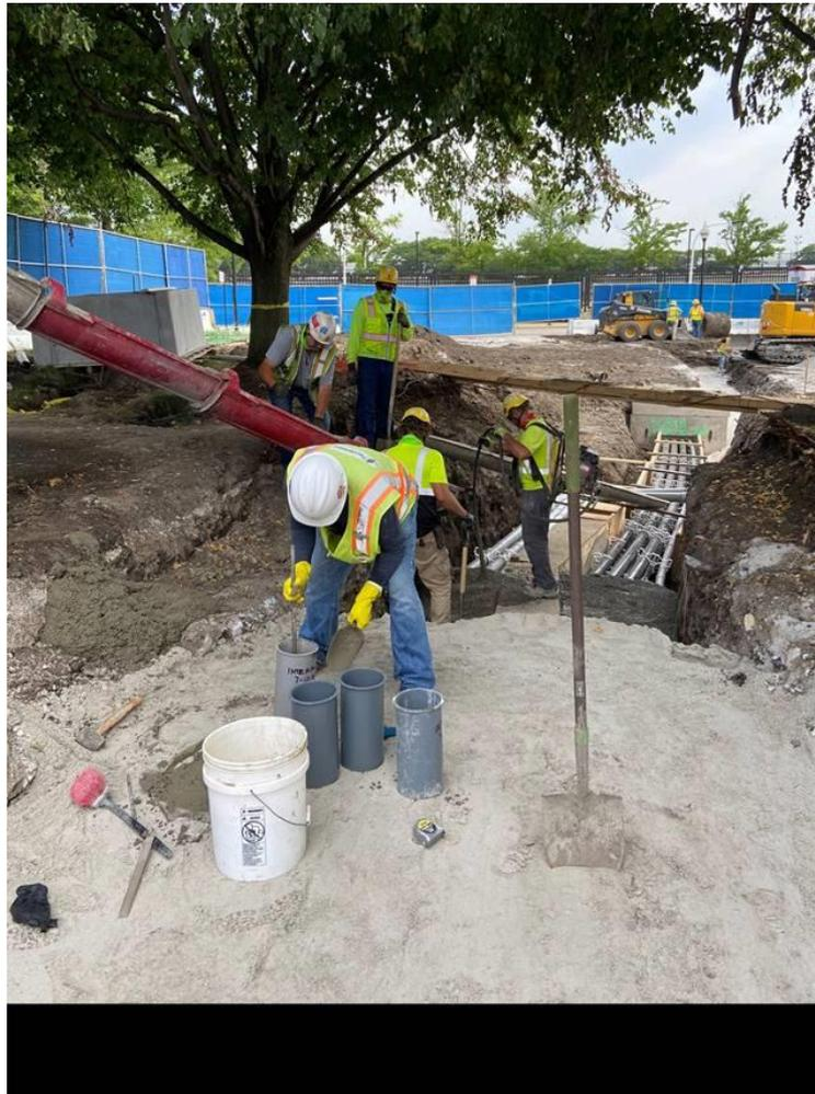
NP – (Left) Conduit from the Vault – (Right) Stubbed up conduit into the Building
