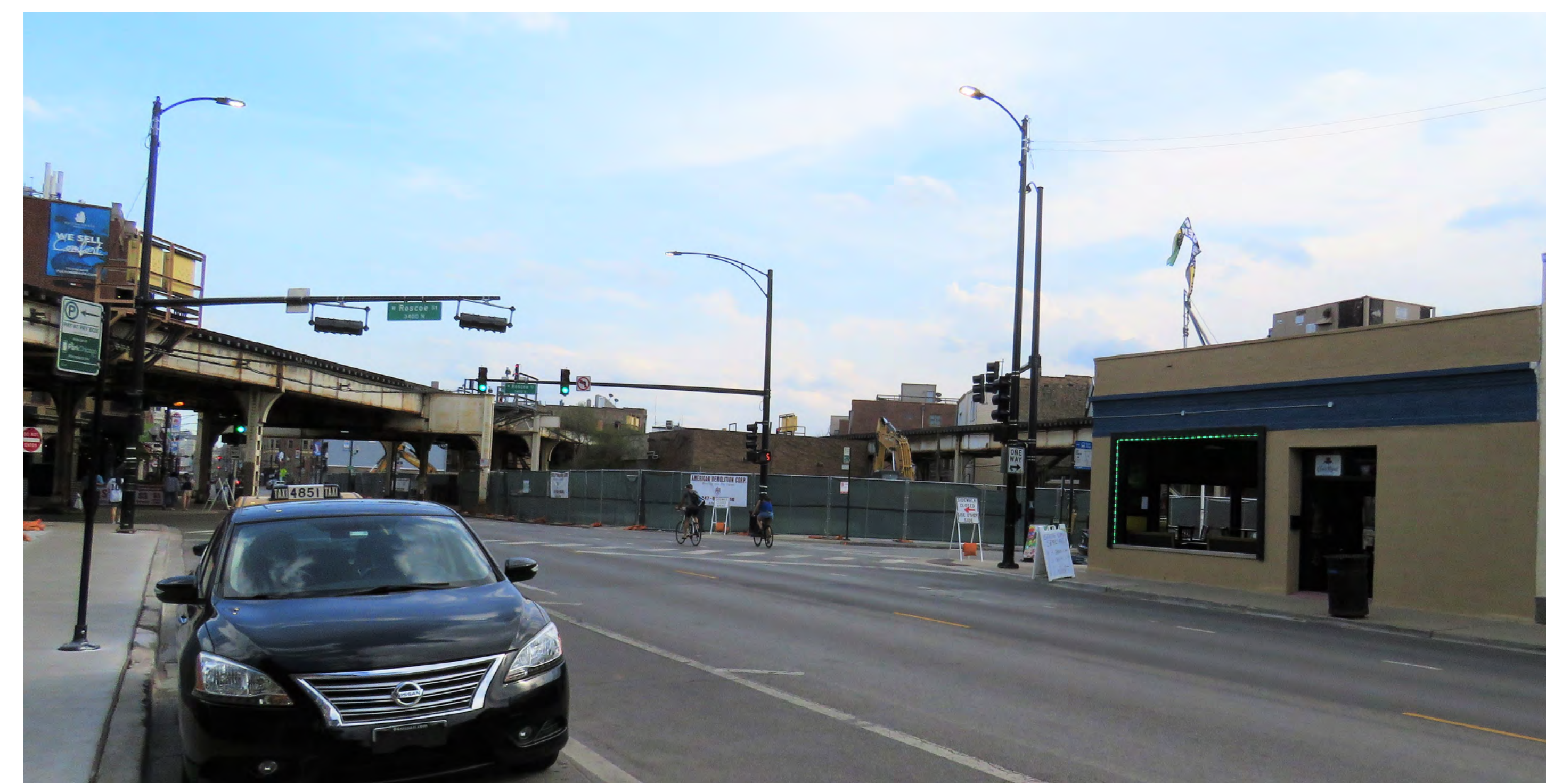
Looking Southwest on Clark Street
