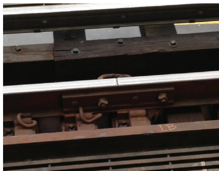
Jointed versus welded rail
