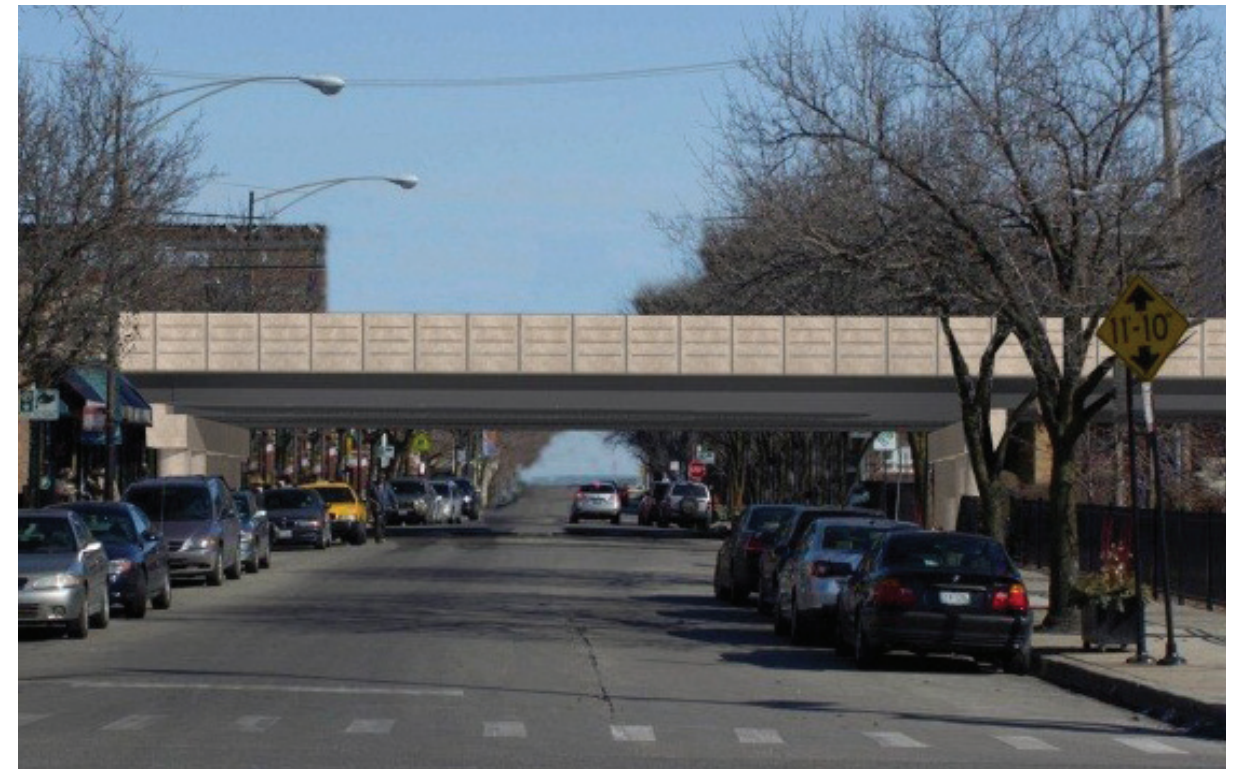
Concept for new viaduct with no columns in the street
