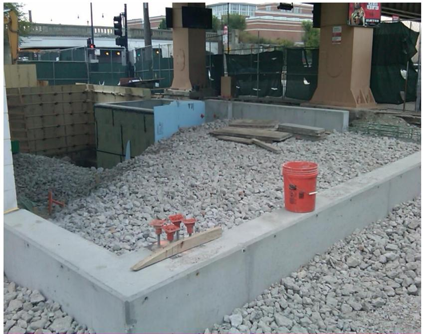
**South, west walls poured. Elevator pit poured as well. Backfilling has begun.**
