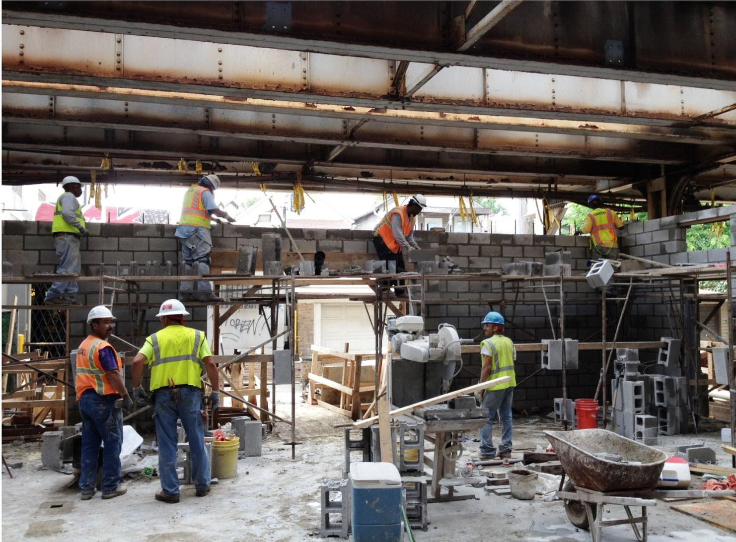
**Armitage Substation: West wall masonry installation**
