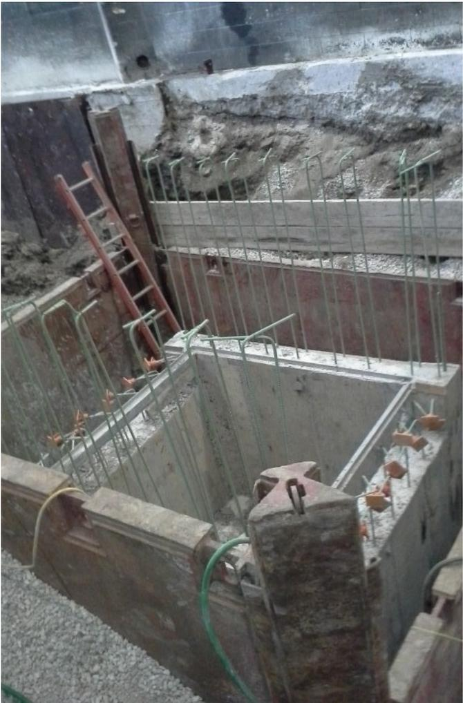
**Sediment Pit for Chassis Wash Foundation Installation –
