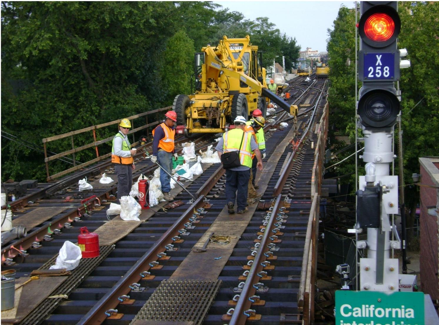
**Installing Running Rail at California Interlocking – WE#9**
