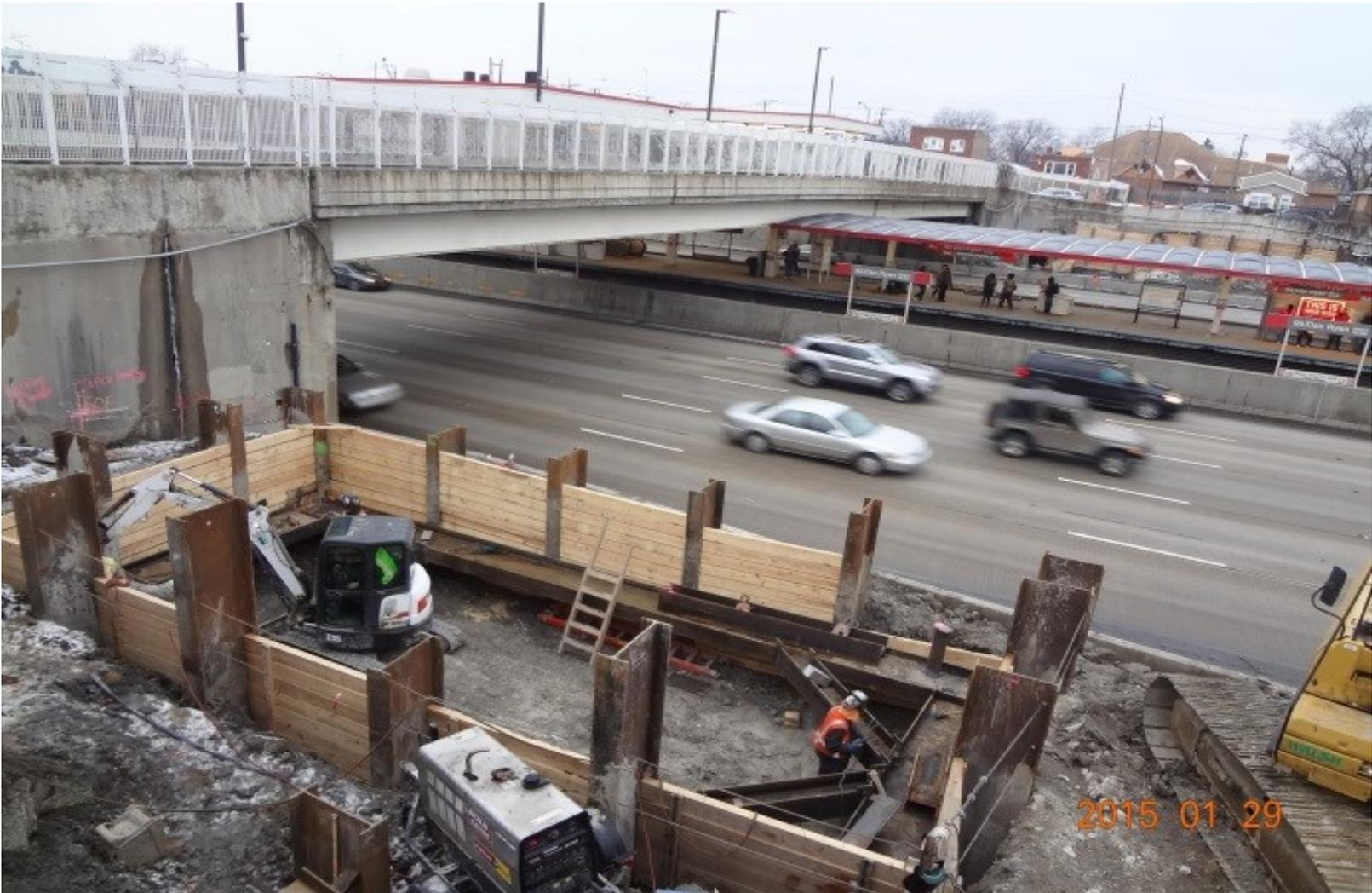
**AP2: Northeast Quadrant (Wall 6) Earth Retention System for Jacking Pit for Fiber Optic and Electrical Ductbank under 95<sup>th</sup> Street**
