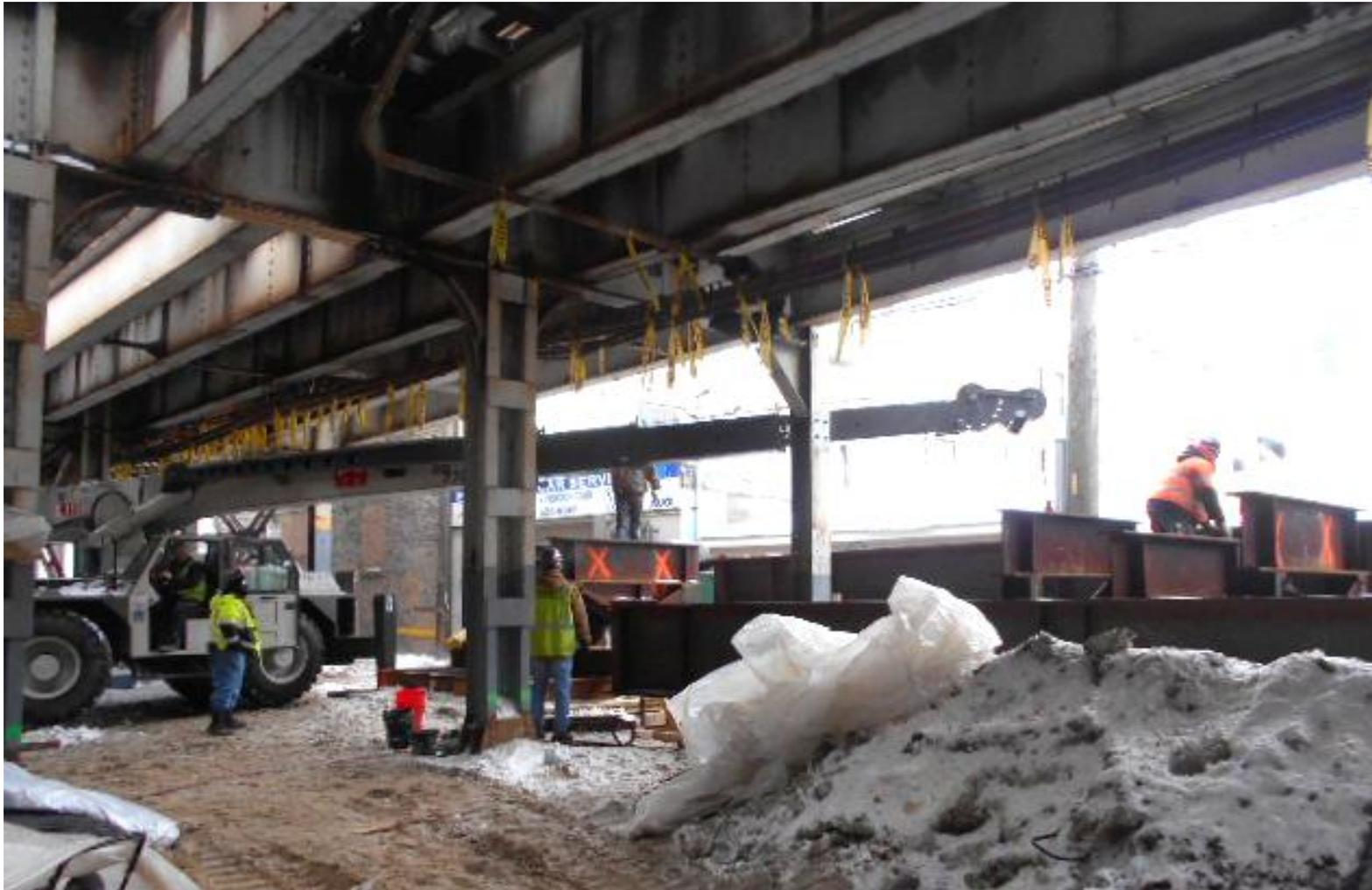
**Armitage Substation: removing shoring from Bent 4069**
