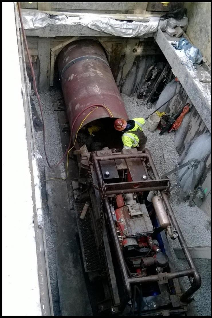
Hill Ductbank: boring north under Hill St. from jacking pit
