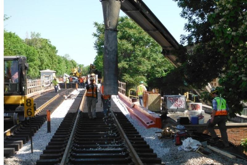
**Bridge Deck Preparation and track installation at Lunt Street Viaduct of the Morse Station**
