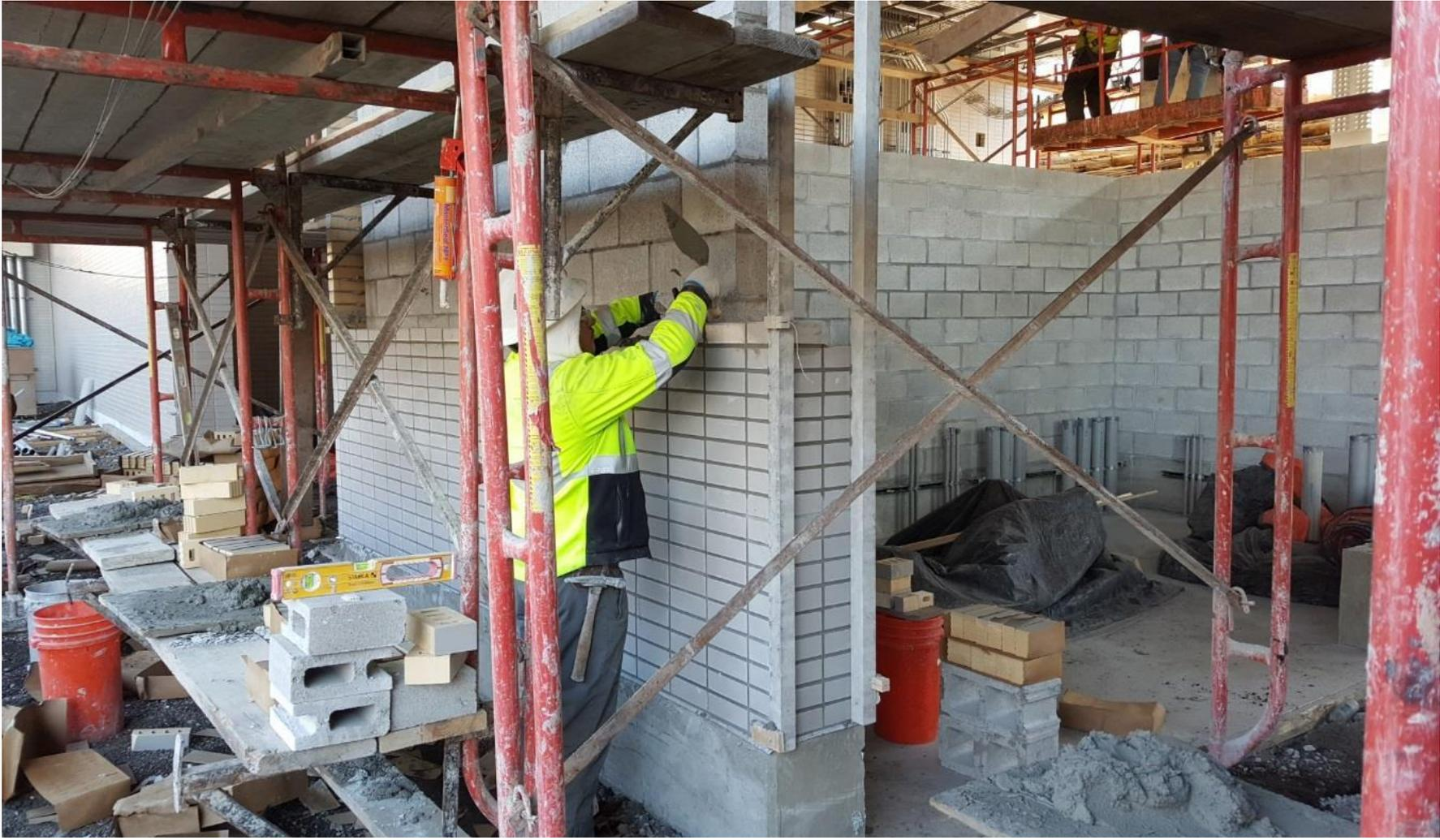
**New glazed tile installation for generator enclosure**
