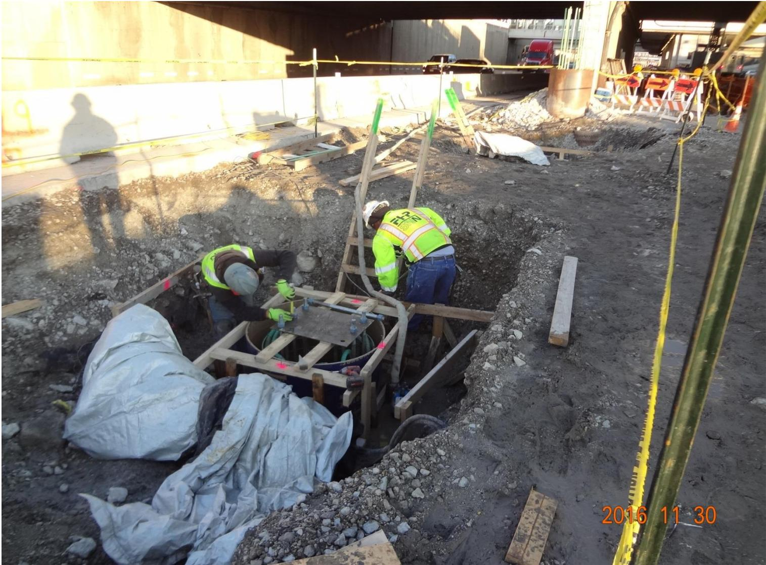
**Forming for west wall caisson cap installation**
