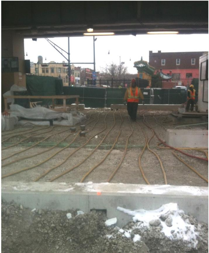
**Underground work complete. Contractor preparing to pour slab.**
