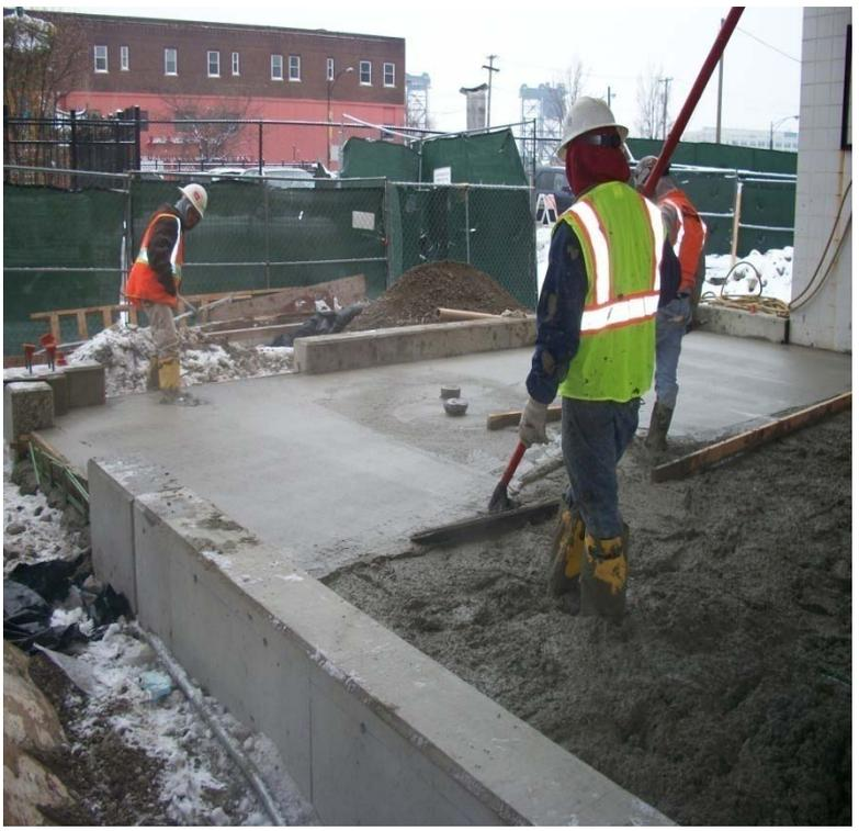
**Station House interior concrete floor slab placement at south end of station.**
