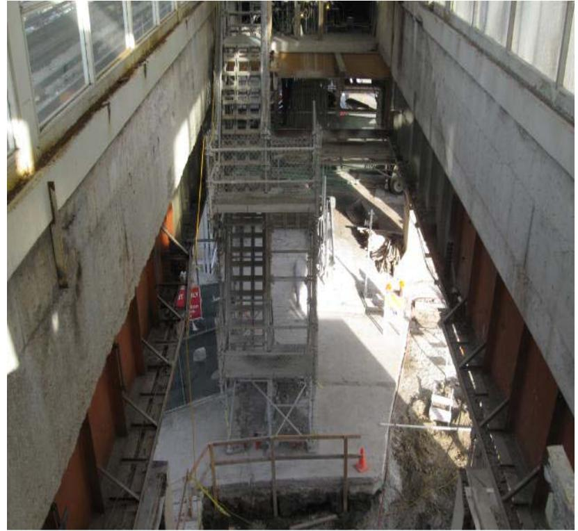
**Detailing of new escalator and stair support steel below platform.**
