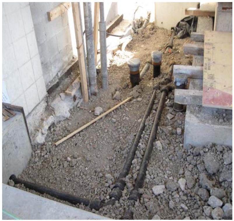
**Underground sanitary plumbing work is complete. Inspected and approved by City of Chicago.**
