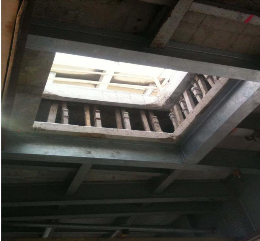
**New platform support steel at location of elevator opening.**
