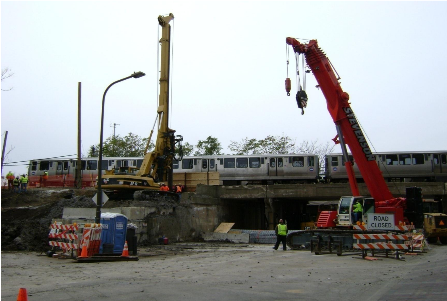
Caisson drilling at Grove
