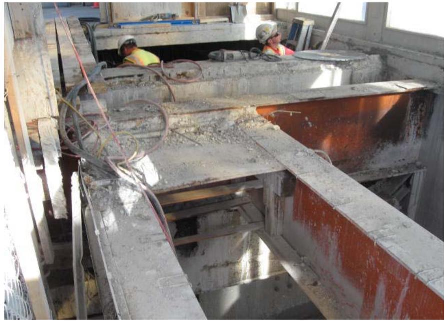
**Platform concrete removal to accommodate new escalator , stair and new walkway to south Cermak.**
