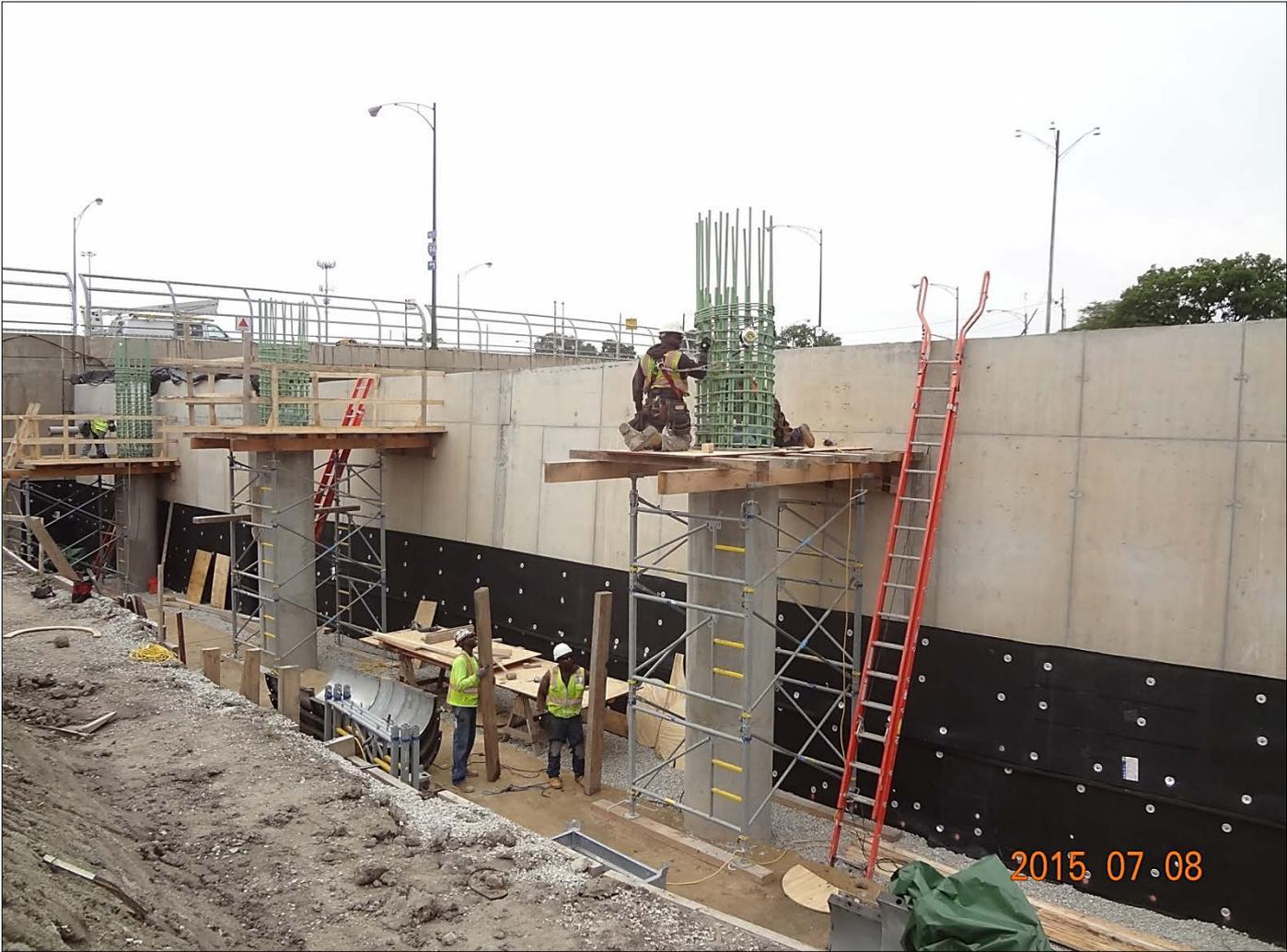
**AP2: Column Rebar Work on Southwest Quadrant (Wall 1)**
