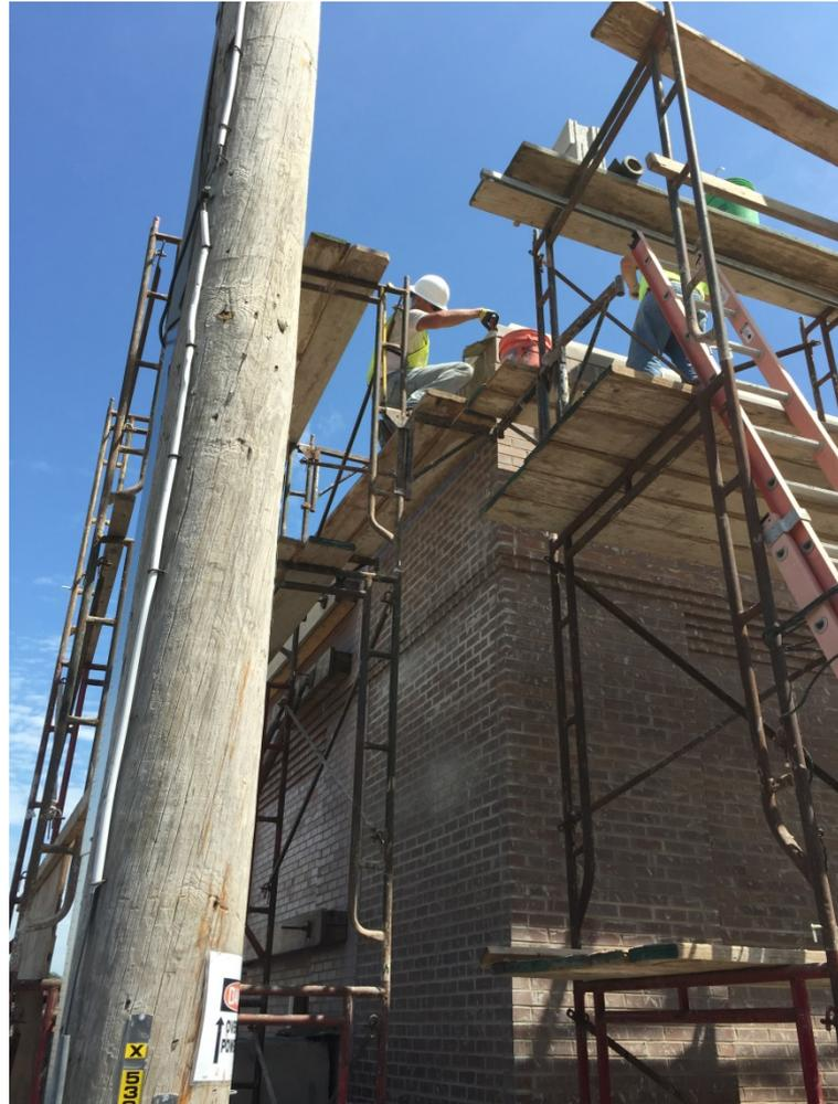
**Kimball Substation: Installation of Roof Coping**
