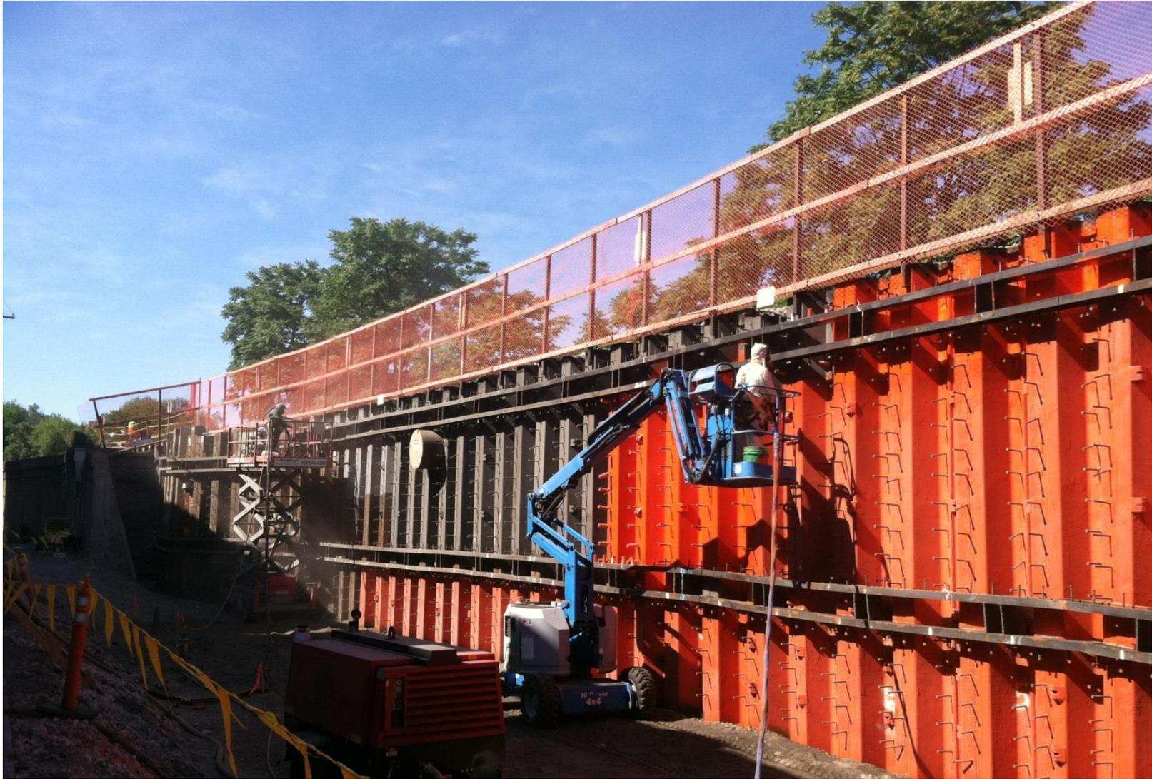
**Contractor sandblasting and waterproofing sheet pile retaining wall at Farwell Substation**
