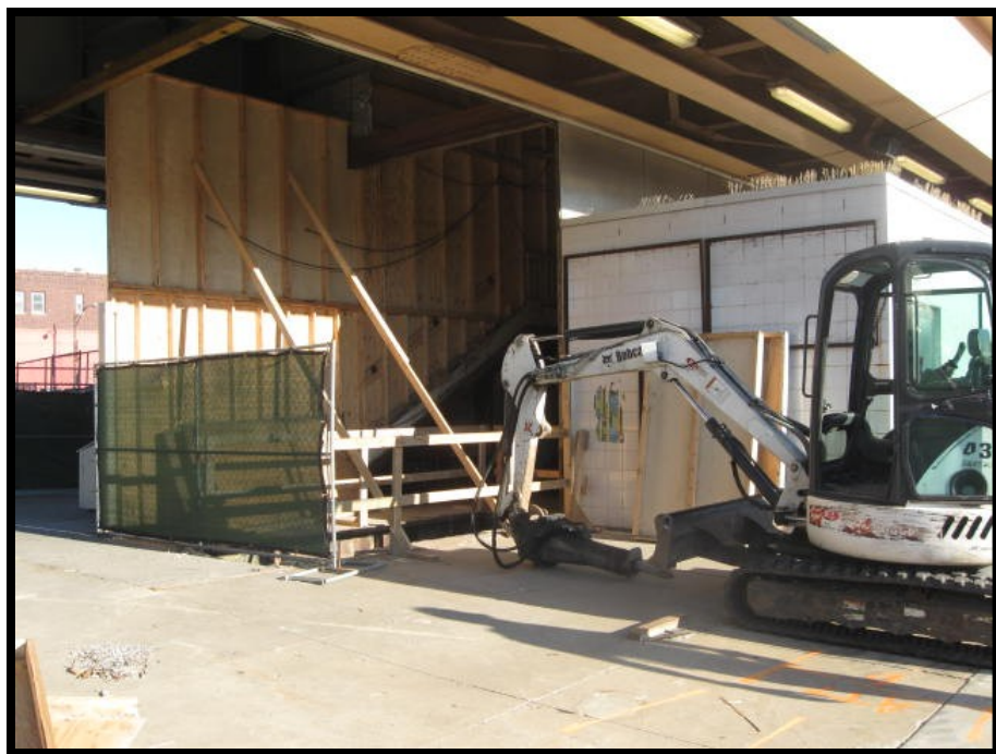
Excavation of damaged escalator's pit began, but has been put on hold due to strike.
