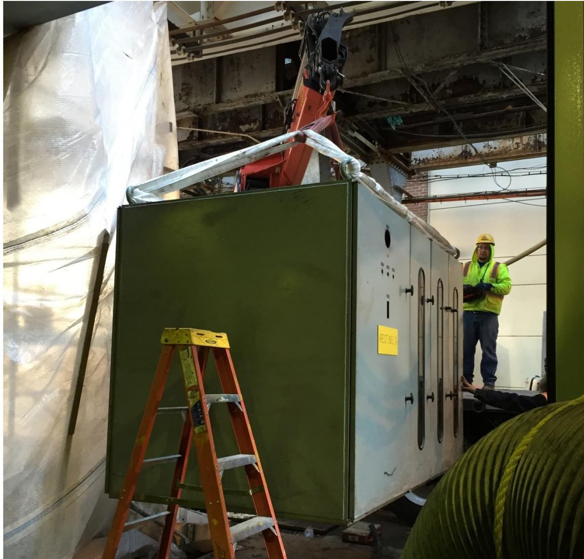
**State Substation: Removal of Existing DC Rectifier**
