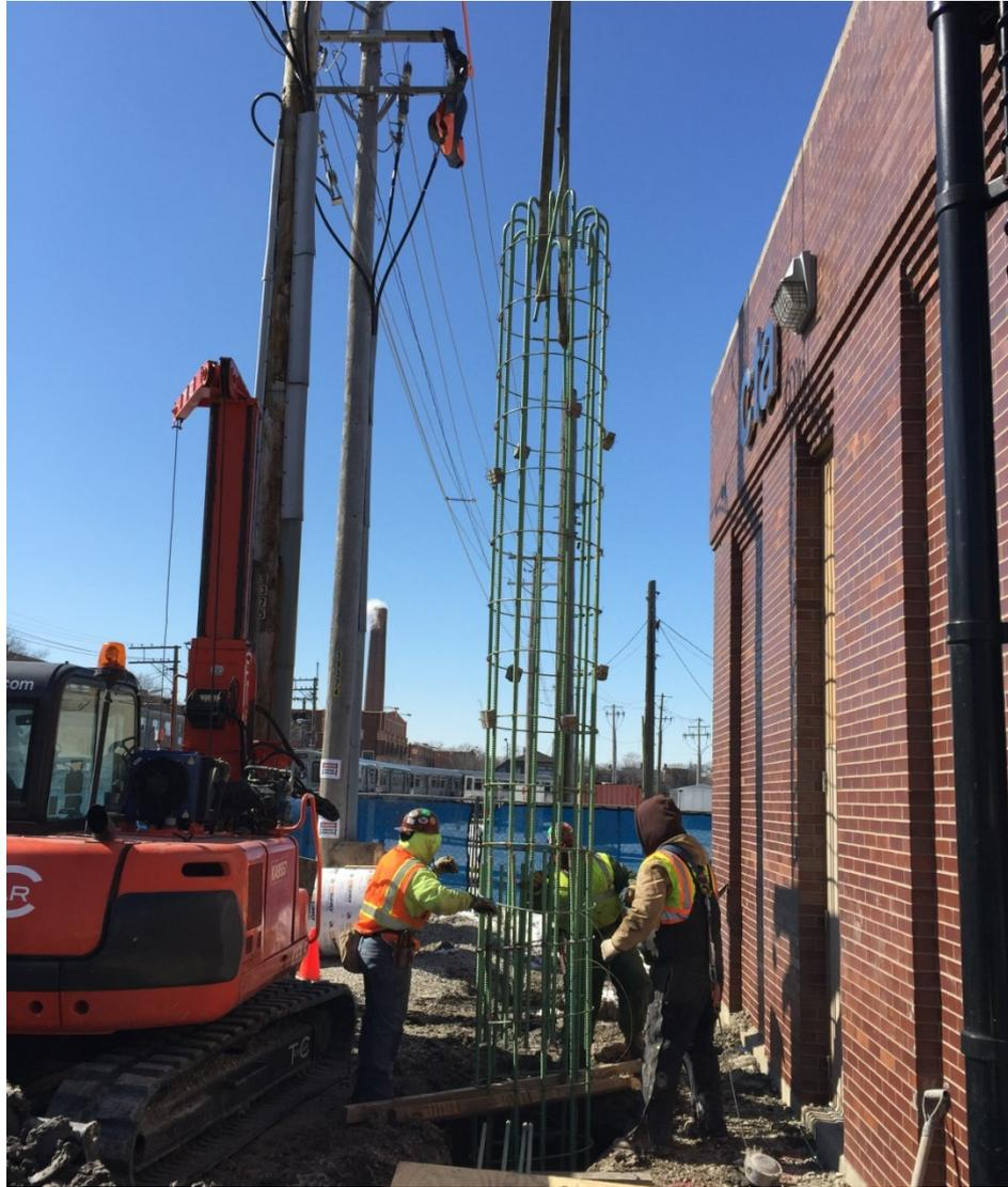
**Kimball Substation: Caisson Installation for New Foundations**
