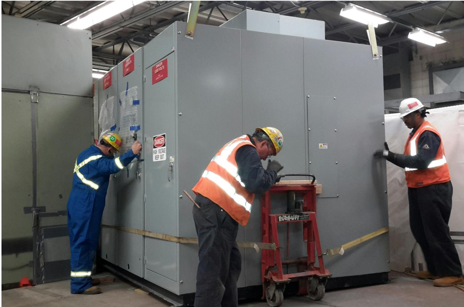
**Princeton Substation: Installing New AC Switchgear**
