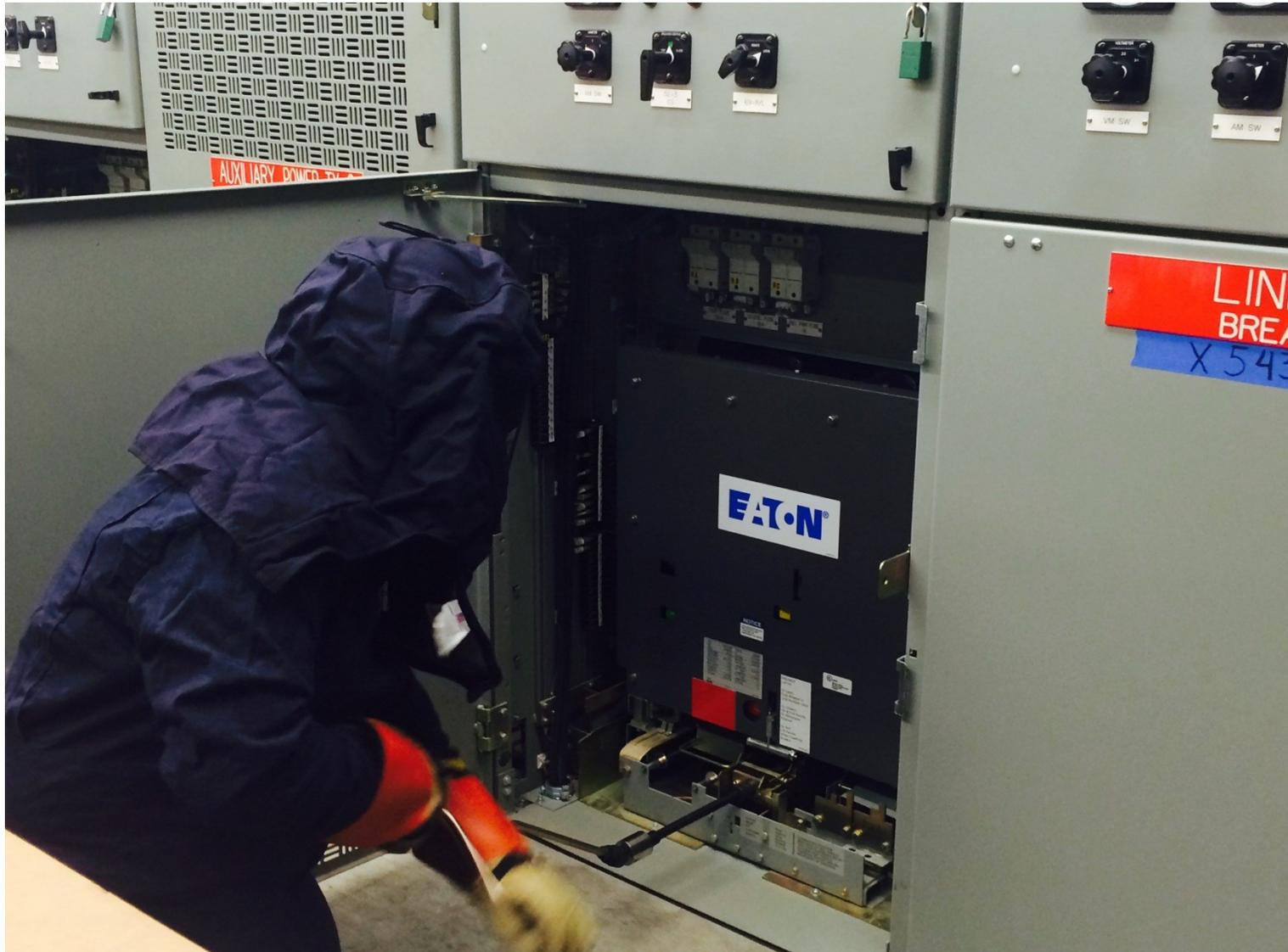
**Armitage Substation: Removing Switchgear with PPE**
