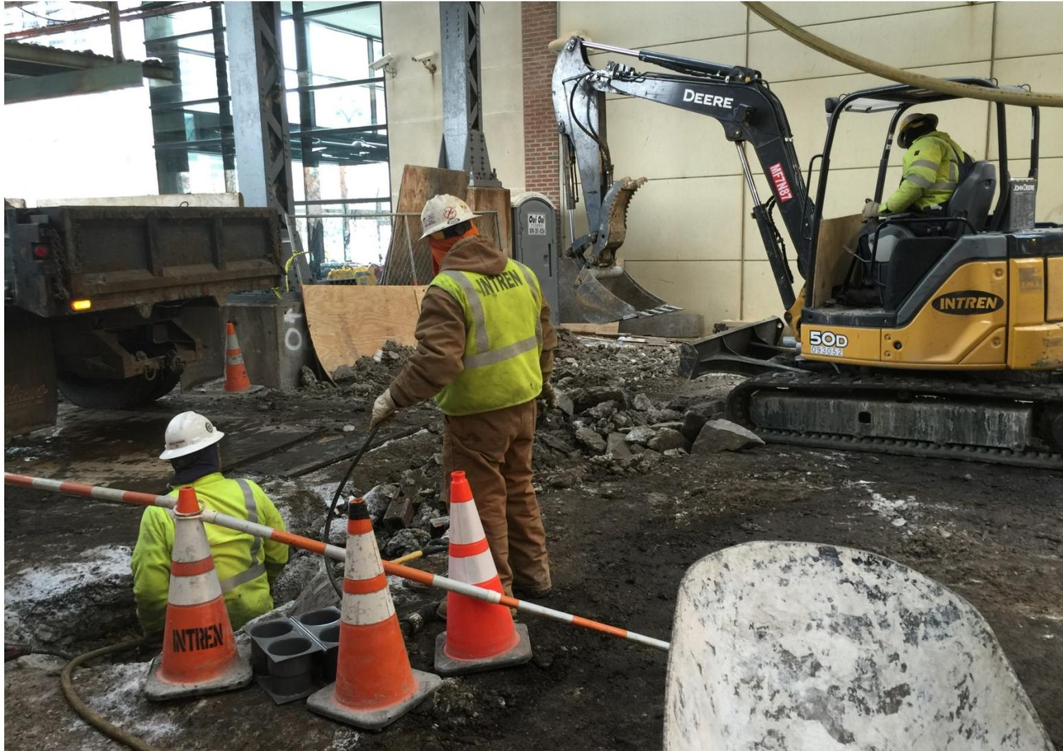
**State Substation: U.G. Installation for New Electrical Service**
