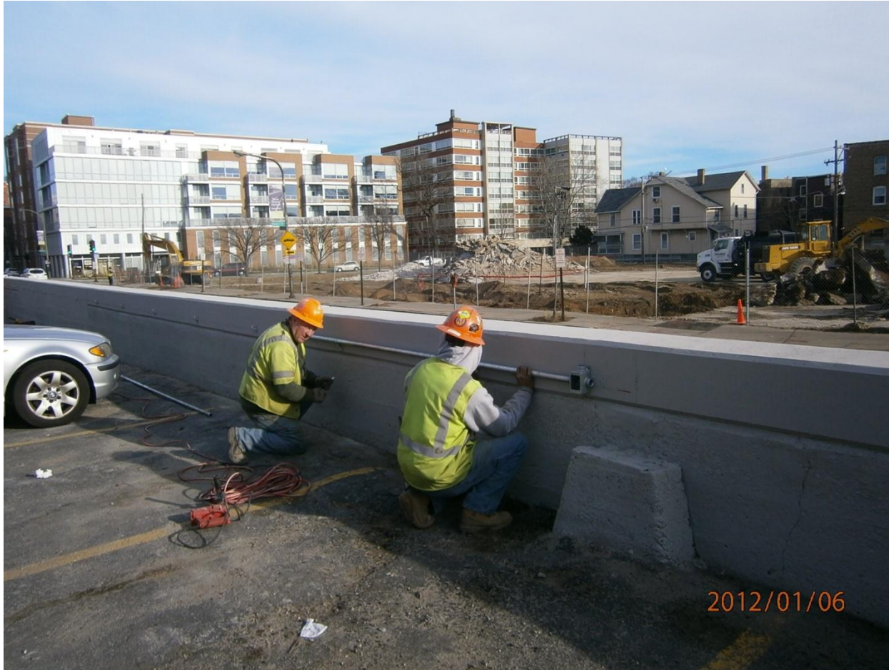
Installing Lighting Conduit at Chicago Retaining Wall
