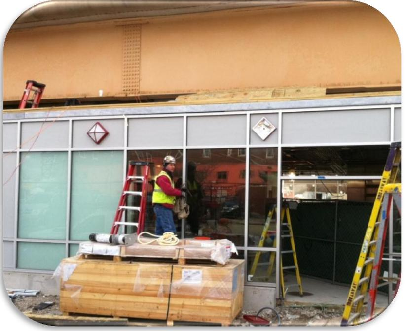
**Station House curtain wall, glass, & exterior station electrical fixtures being installed.**
