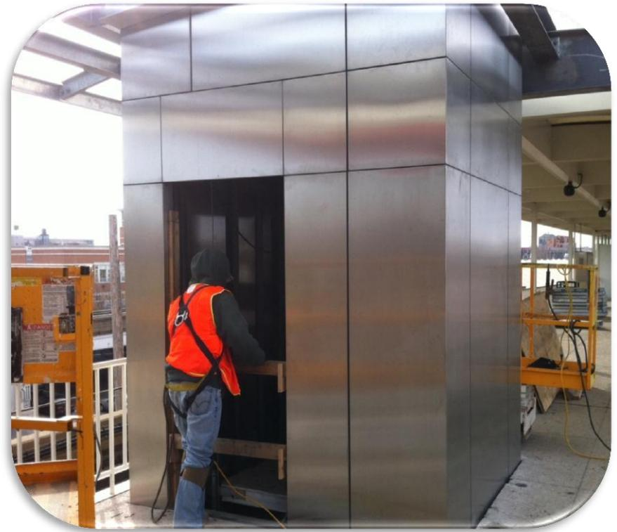
**Elevator exterior tower & panels installed.**
