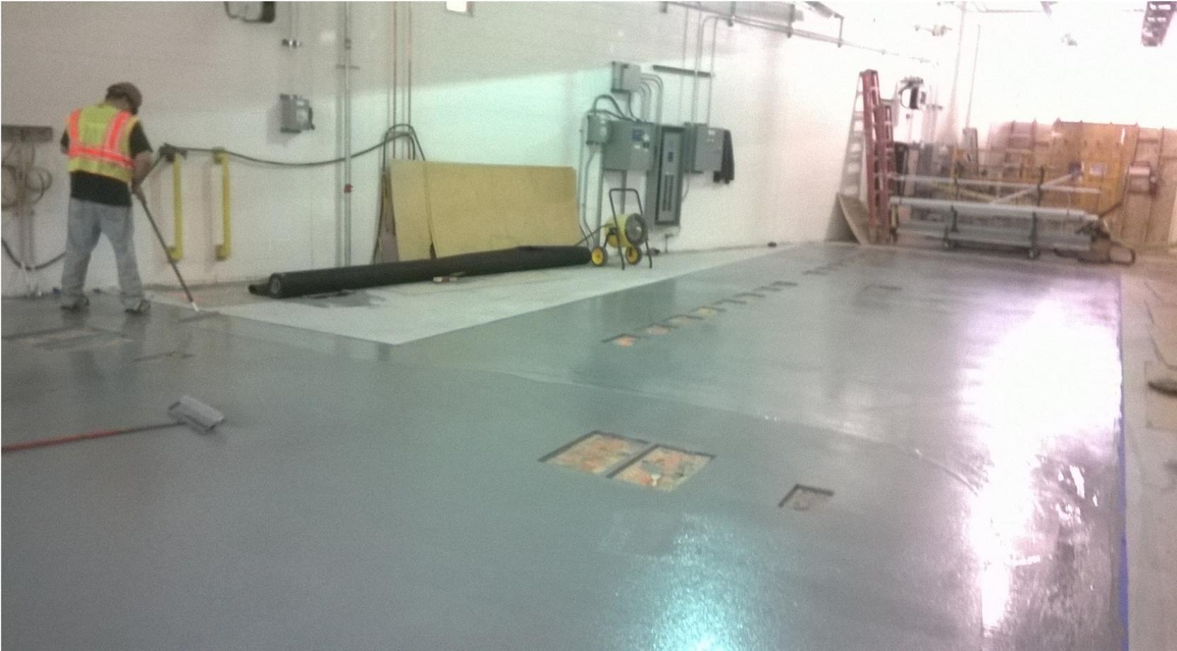
Hill Substation: Interior Dielectric Floor Installation
