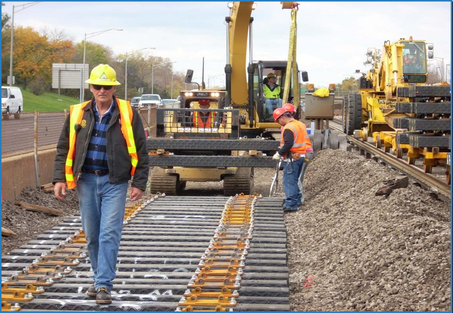
New plastic ties being installed on the O'Hare Branch
