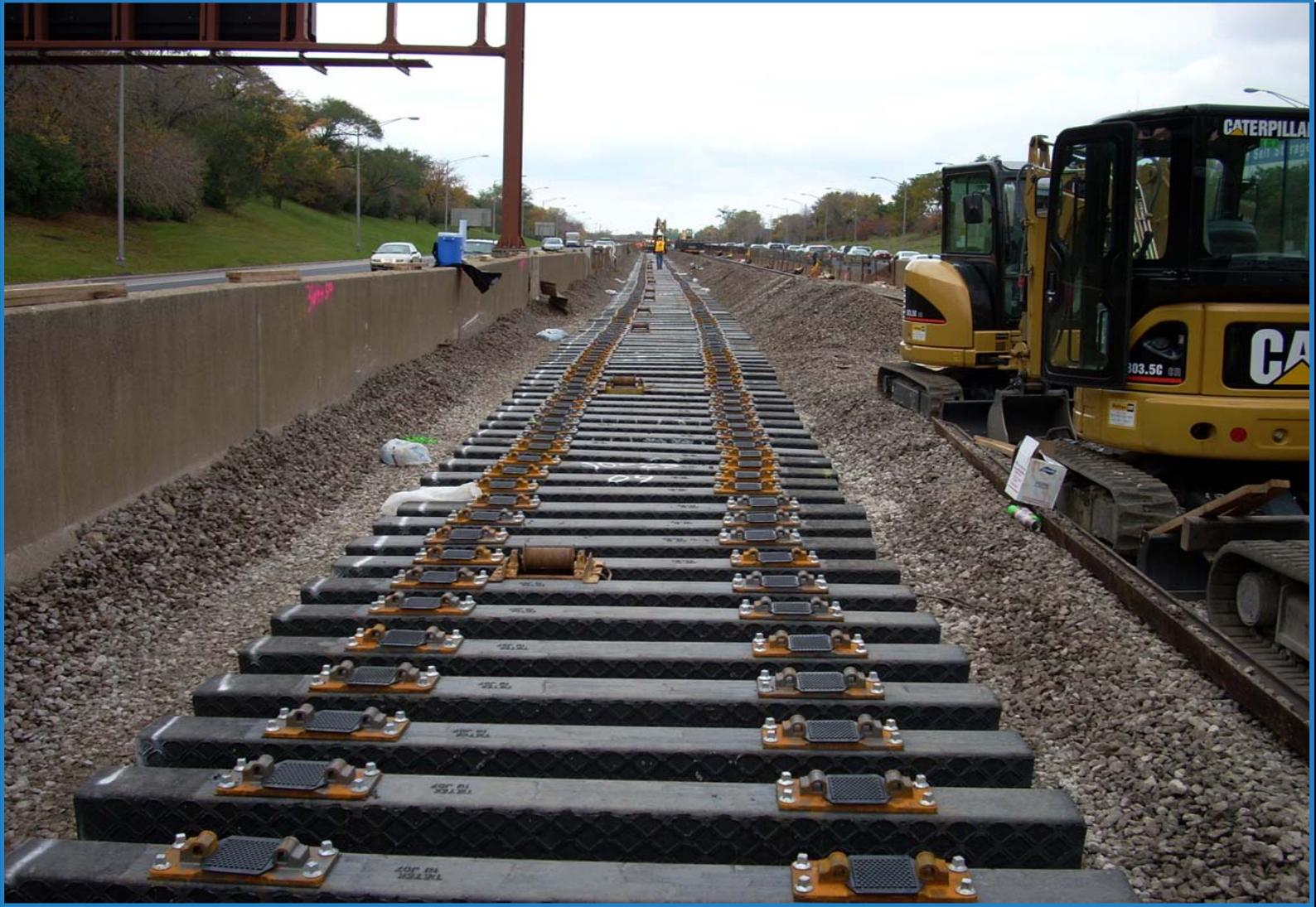
New plastic ties installed on O'Hare Branch
