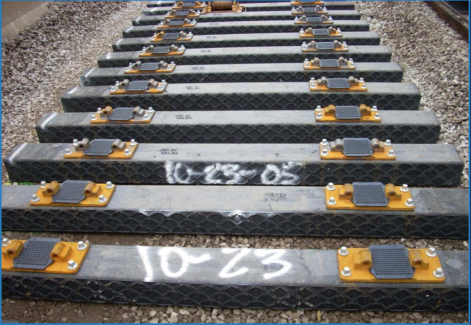
New plastic ties installed on O'Hare Branch
