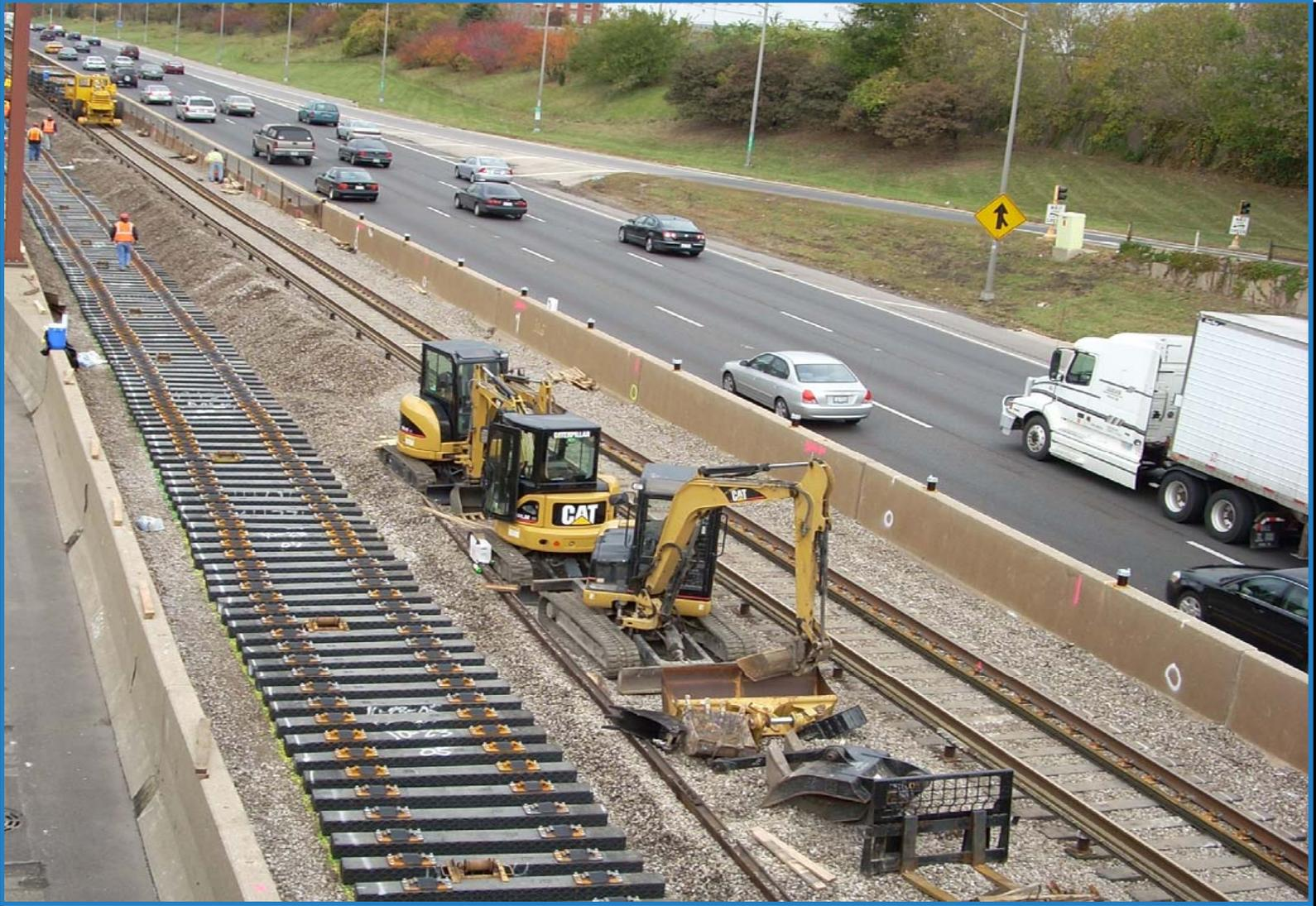
New plastic ties installed on O'Hare Branch
