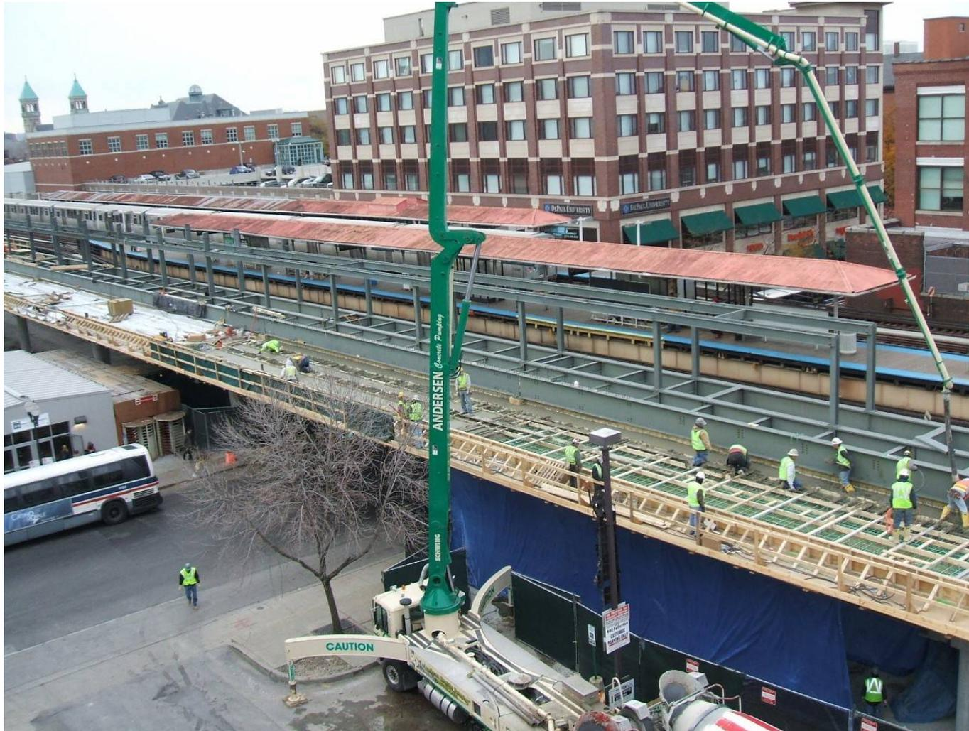
Pouring new concrete track bed at Fullerton
