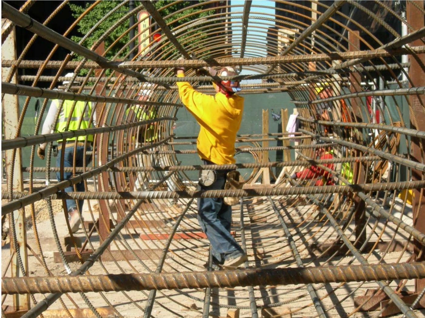
Assembling of caisson rebar frames
