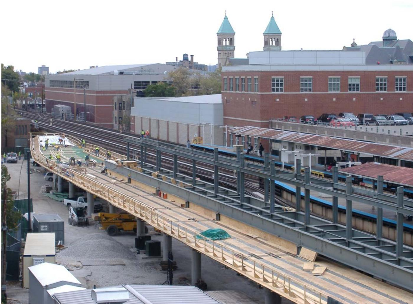
Fullerton Station forming for concrete decking and platform steel
