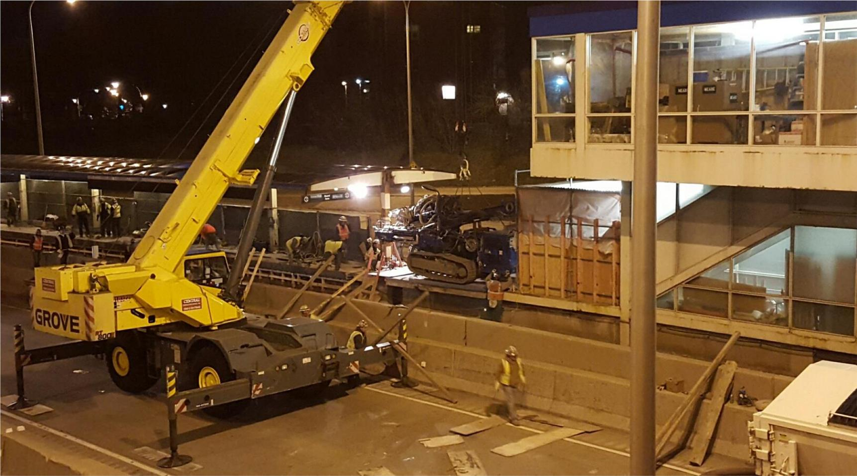
**Addison placement of micro pile rig for new staircase**
