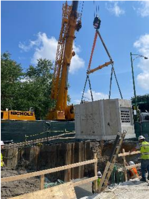
Ductbank Vault Install at Barry
