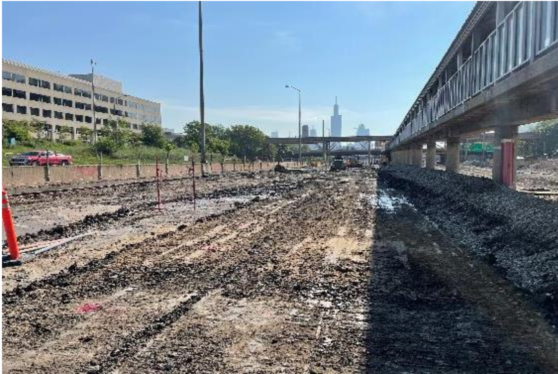
Mass Excavation & Grading by IMD Station
