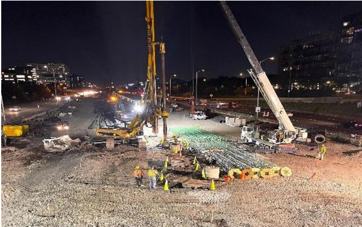
Cassions and Deep Foundations at Racine
