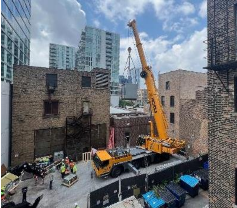
Equipment Installation at Haymarket
