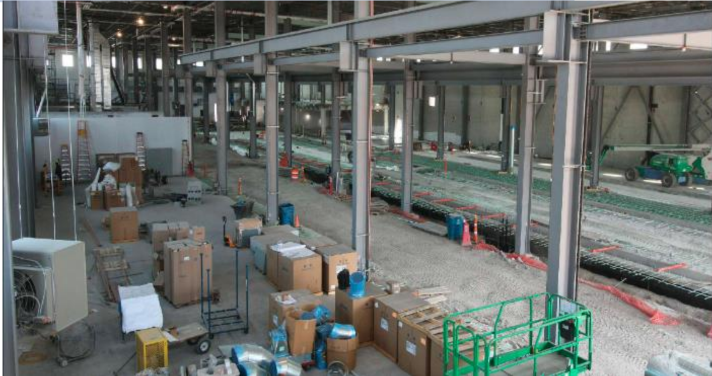
Building Interior – Looking Northeast
