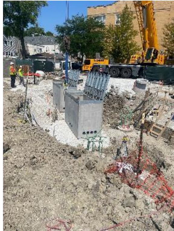
Ductbank Vault Install at Barry
