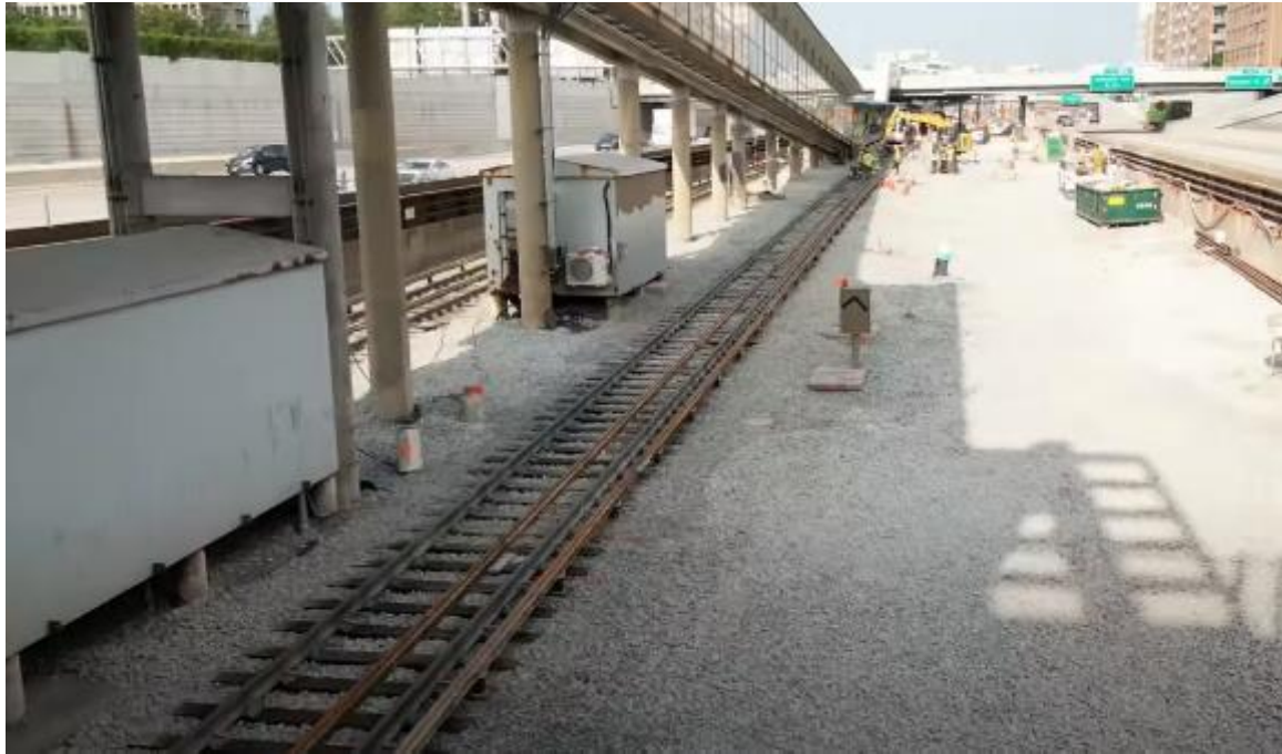
Stage A Completion
