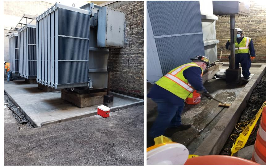
Excavating Soil & Cleaning Existing Concrete Pad at Franklin Substation
