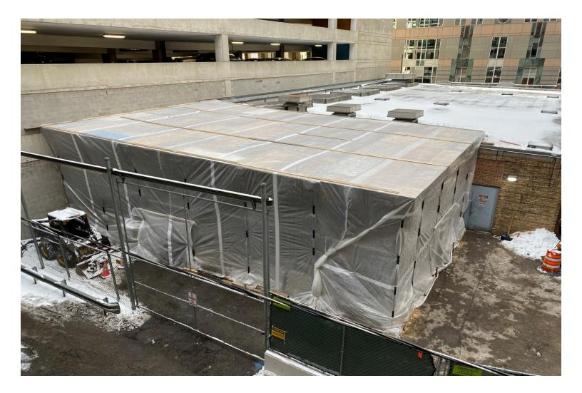
Completed a Temporary Enclosure Around All Transformers at Franklin Substation
