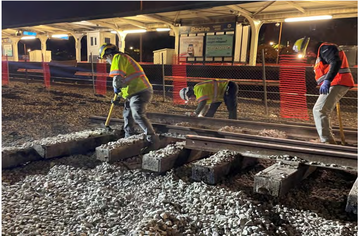
Racine Siding Track Demolition
