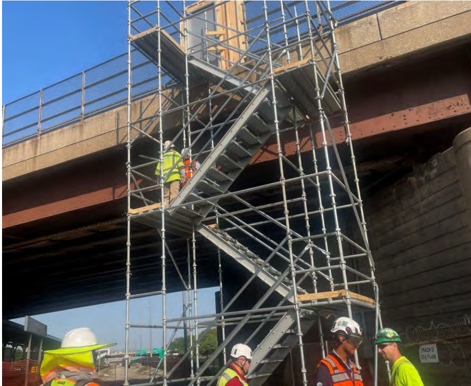
Installation & Inspection of Stair Tower at Ogden
