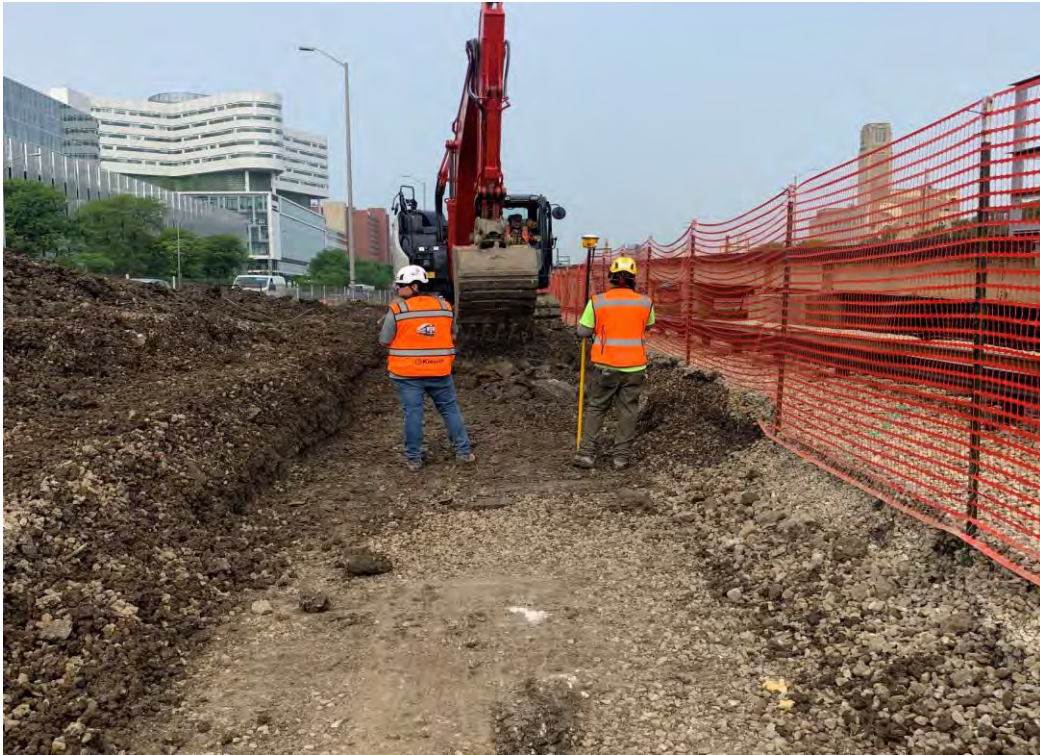
Excavation & Grading South of Loomis Incline
