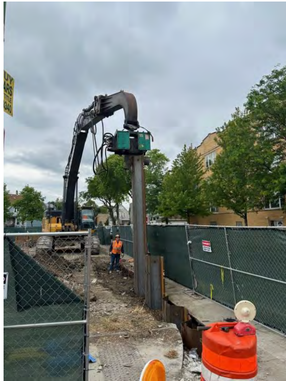
Earth Retention System Installation at Barry
