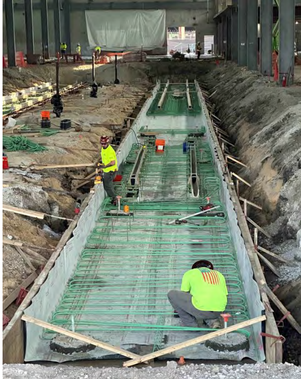
CAP – Installing Trench Drains
