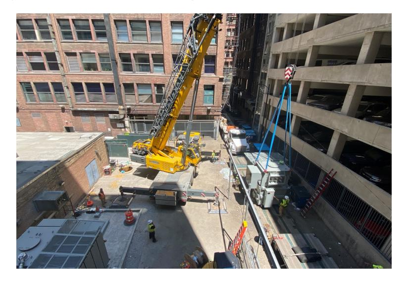
Lifting and Placing New Transformer 3 at Franklin Substation
