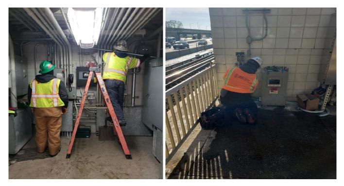
Transformer & conduit install wire at 63rd electric room
