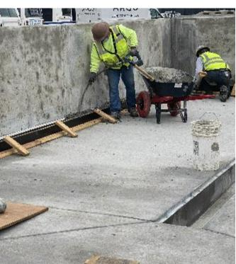
Exterior wall forms stripped and floor poured
