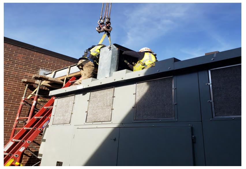
Mounting Anode Bus Box Up for Transformer#1 at Edmunds Substation
