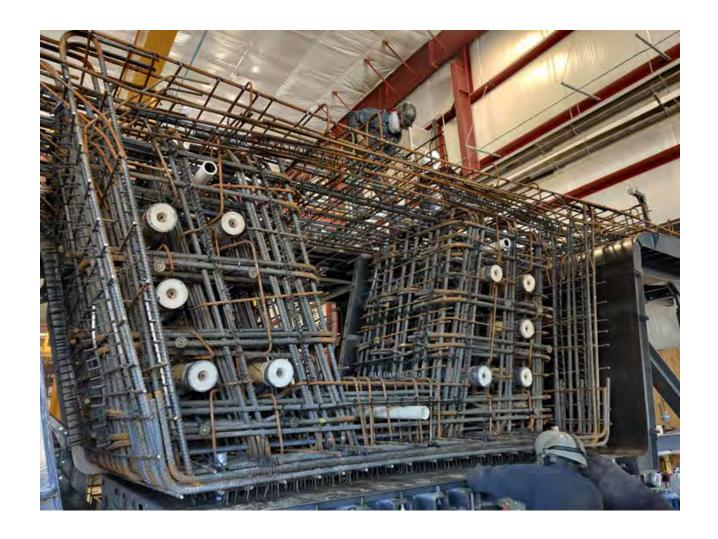
Lawrence to Bryn Mawr Modernization Box Girder End Segment Rebar Cage Installation
