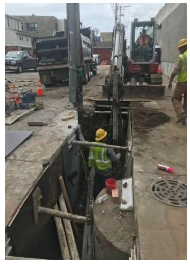
Water main installation by CDWM-Water on Sheffield (left) and ComEd trench excavation and shoring in east alley south of Lawrence (right)
