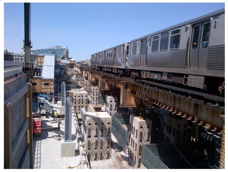
New track 2 concrete pedestals/columns and shoring
