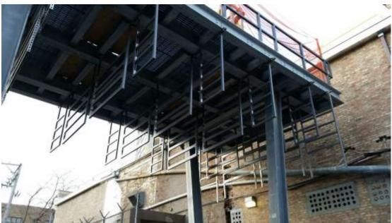
Di-electric Floor Installation (Left) and Cable Bridge Installation (Right)
