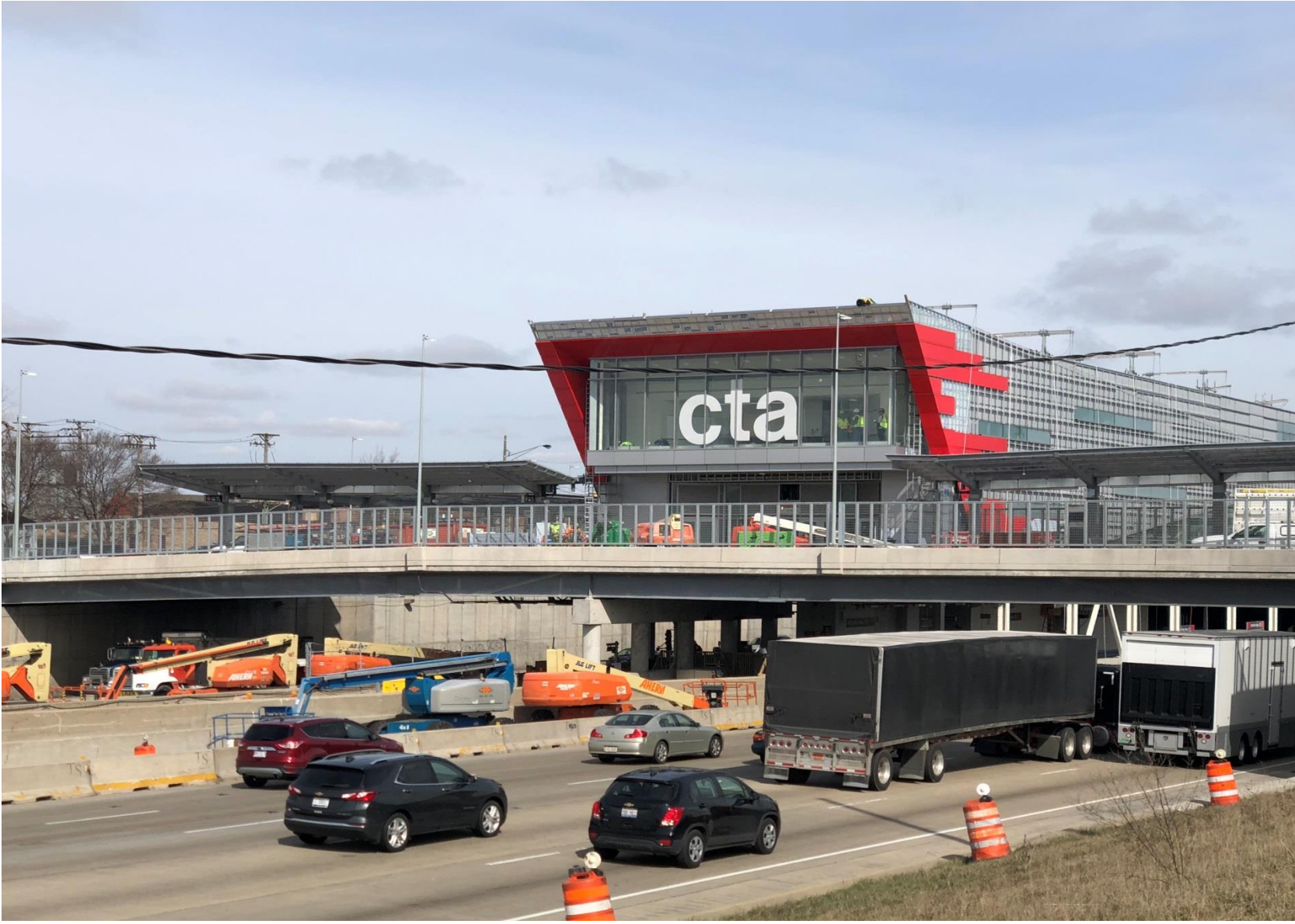
South Terminal: South Bus Bridge
