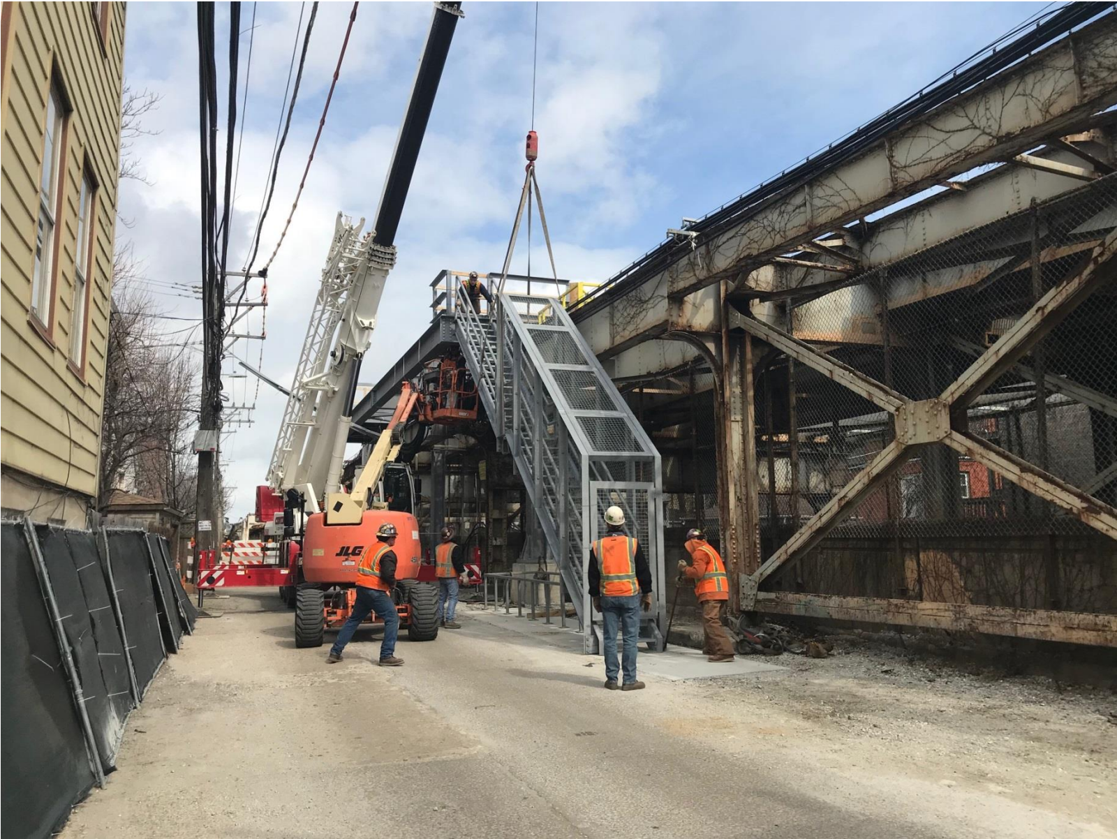
Setting Willow Relay House Access Stair
