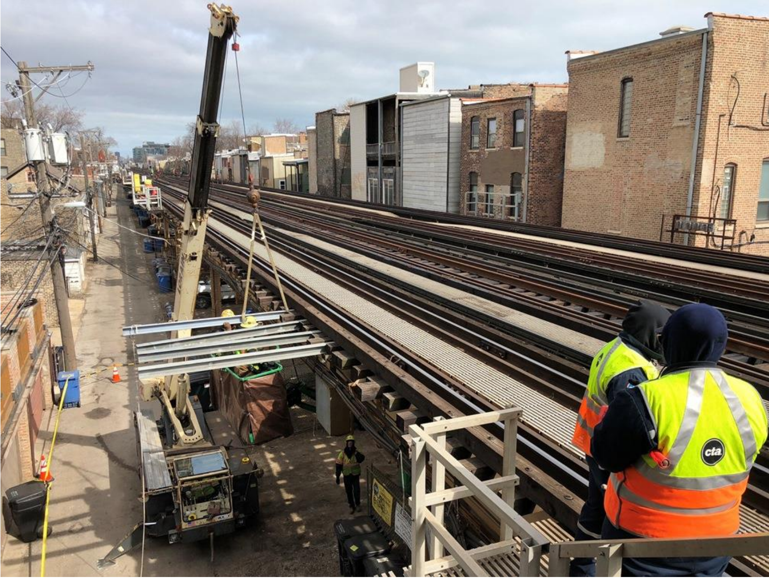
Setting Bond Platform Steel
