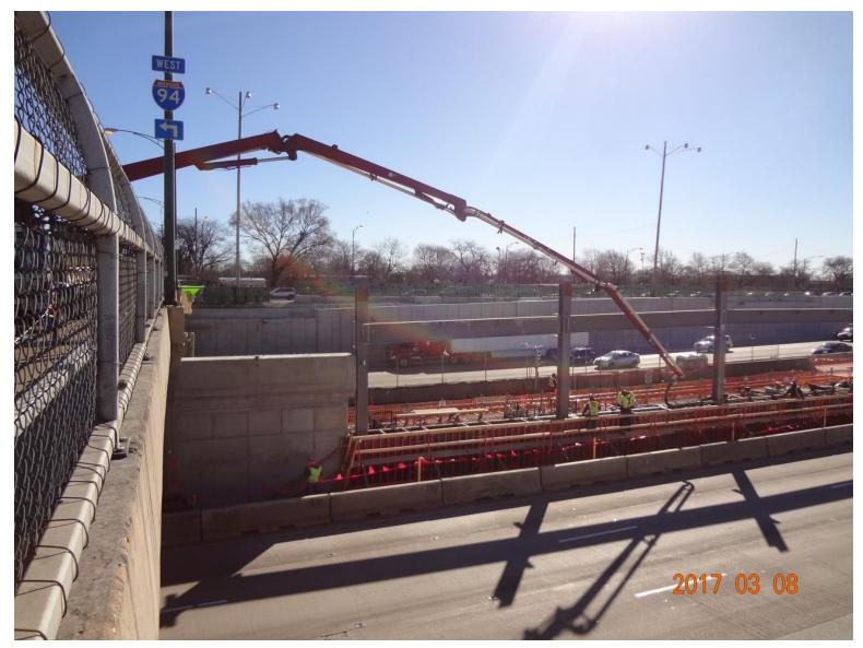
95<sup>th</sup> Bridge Pier Extension Complete, West Side Barrier Wall Concrete Pour
