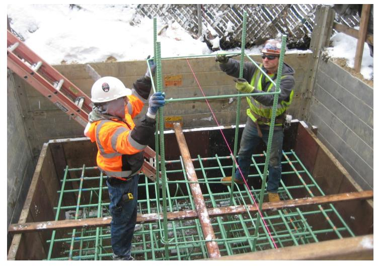
Installation of signal house foundation rebar at Cleveland
