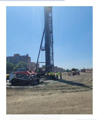
**Pile Drilling Rig**
