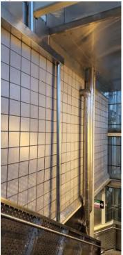
Morgan/Green - Water damage & mitigation. Removal of ceiling and installation of new gutters. Ceiling to be replaced
