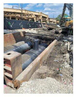
Installing 84" CMP Stormwater Pipe
