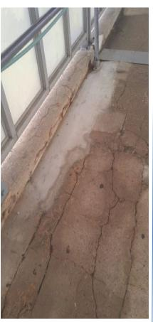
Western (Blue Line Congress) Repair Arears of Loose & Spalling Concrete of the Ramp
