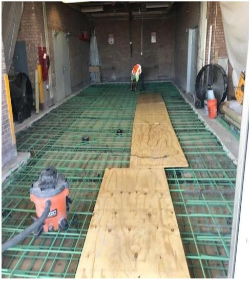
Concrete floor demolition on penthouse level and Reinforcement Bar installation prior to concrete pour
