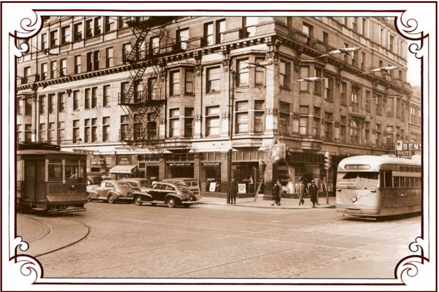
In this post World War II view, a southbound #22 Clark-Vincennes streetcar on its way Downtown meets an eastbound Chicago Avenue streetcar on its way to Navy Pier. Cars 277 and 4280 were both built by the Pullman Company, but 40 years apart. The change in technology and aesthetics is evident.
