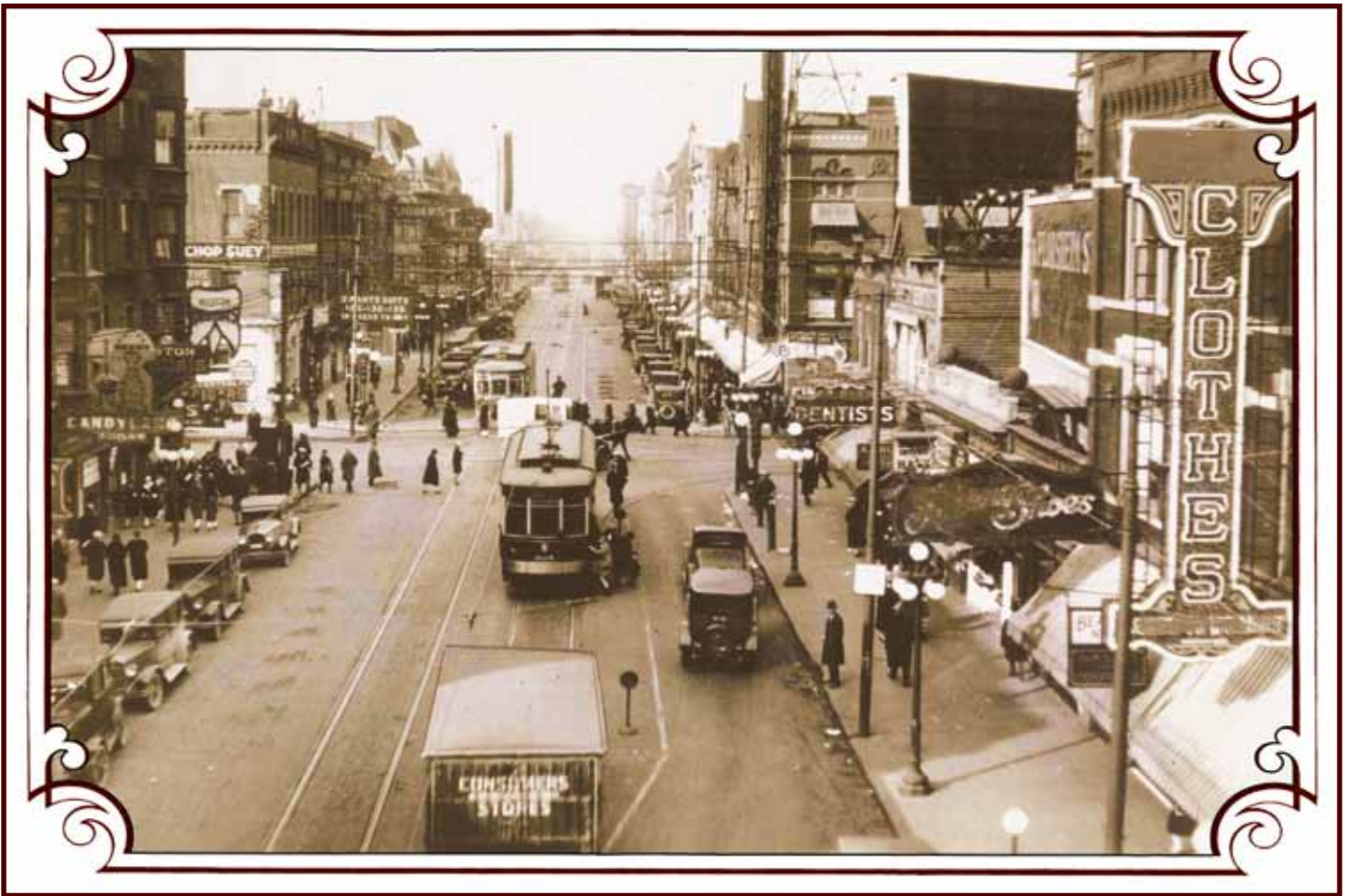
There's no shortage of streetcar service in this view taken from Englewood's Halsted 'L' station on March 10, 1928, looking north on Halsted. This vantage point shows a bustling and vibrant business district replete with clothing and shoe stores, furniture stores, candy shops, restaurants, and assorted specialty shops.
