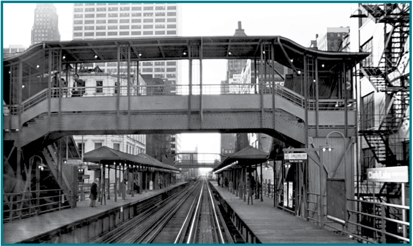
This is a train's-eye view looking west along the Loop Elevated above Lake Street of the original Clark/Lake elevated station as it looked shortly before construction of a replacement station began in 1988. Originally opened in 1895, this station and State/Lake were built by the Lake Street Elevated and actually predated the Loop 'L' by a few years, being incorporated into the downtown quadrangle in 1897. Almost everything seen in this photo is gone today, as this station has been replaced with a new, modern, ADA-accessible station with direct connection to the subway below it.
