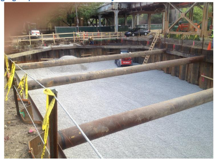
Hill worksite, ERS and CA-7 stone, preparation for foundation installation
