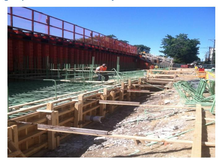
**Contractor installing reinforcing bars for foundation installation at Farwell Substation**
