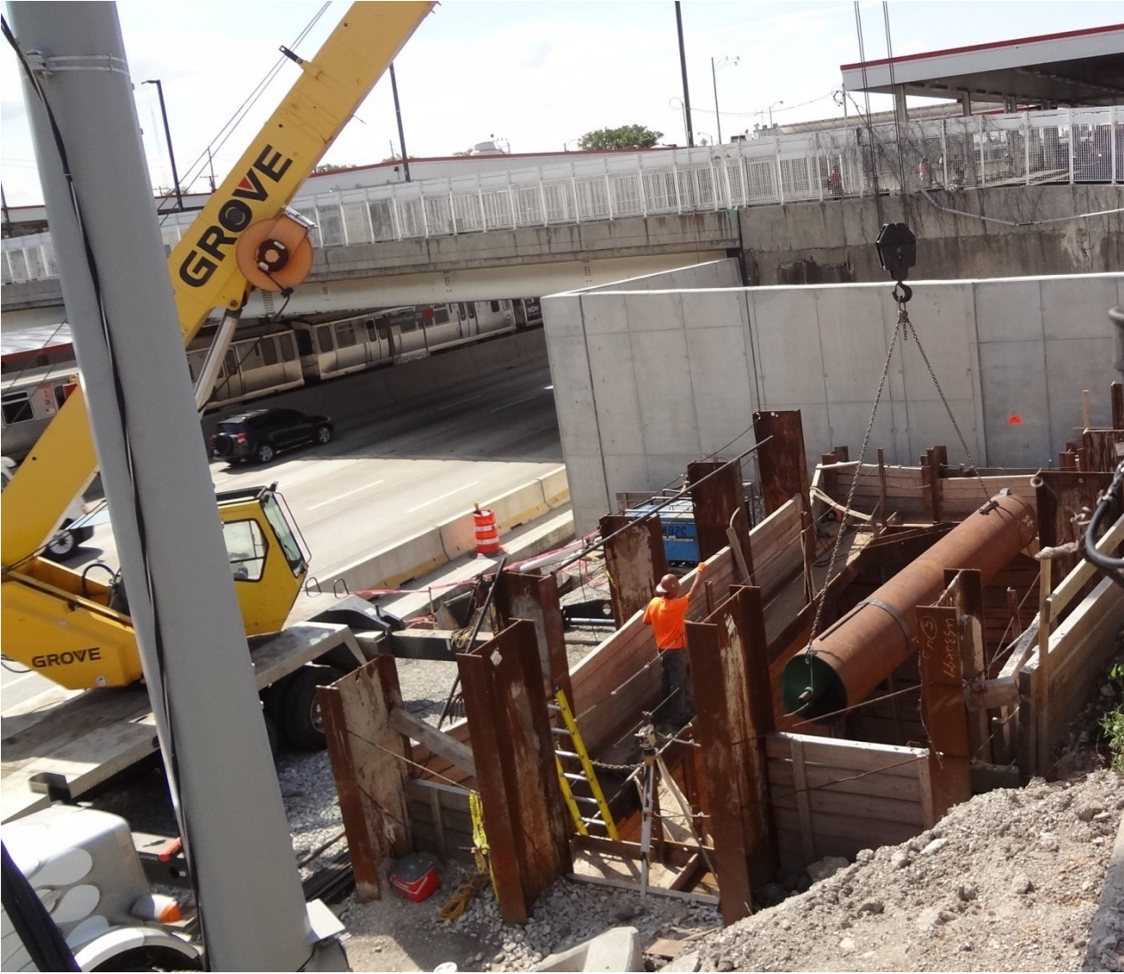
AP2: Jack and Bore Casing Installation on East Side (Wall 2)
