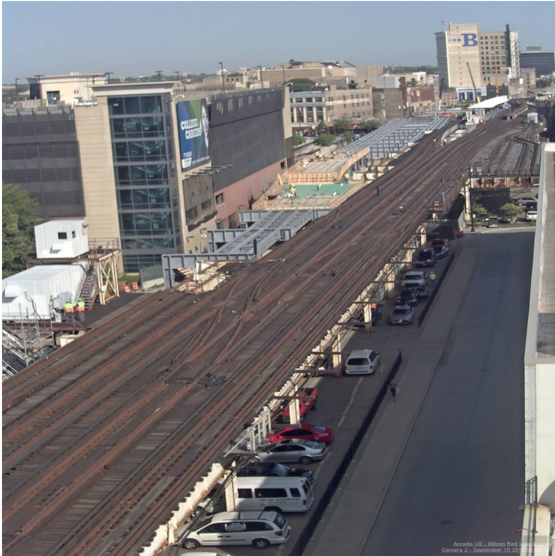
New Track 1 structure
