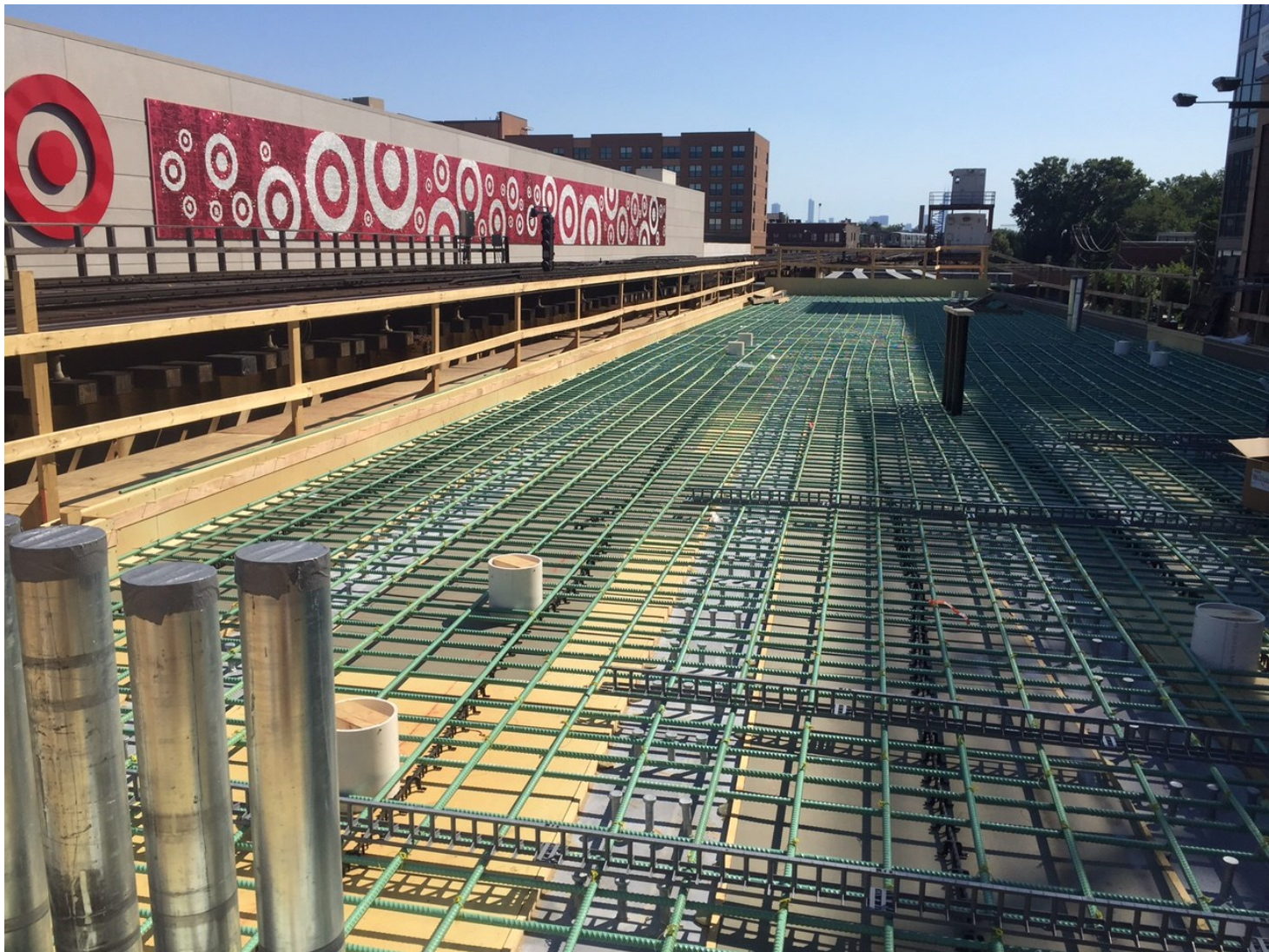
New track 1 deck framing/rebar installation
