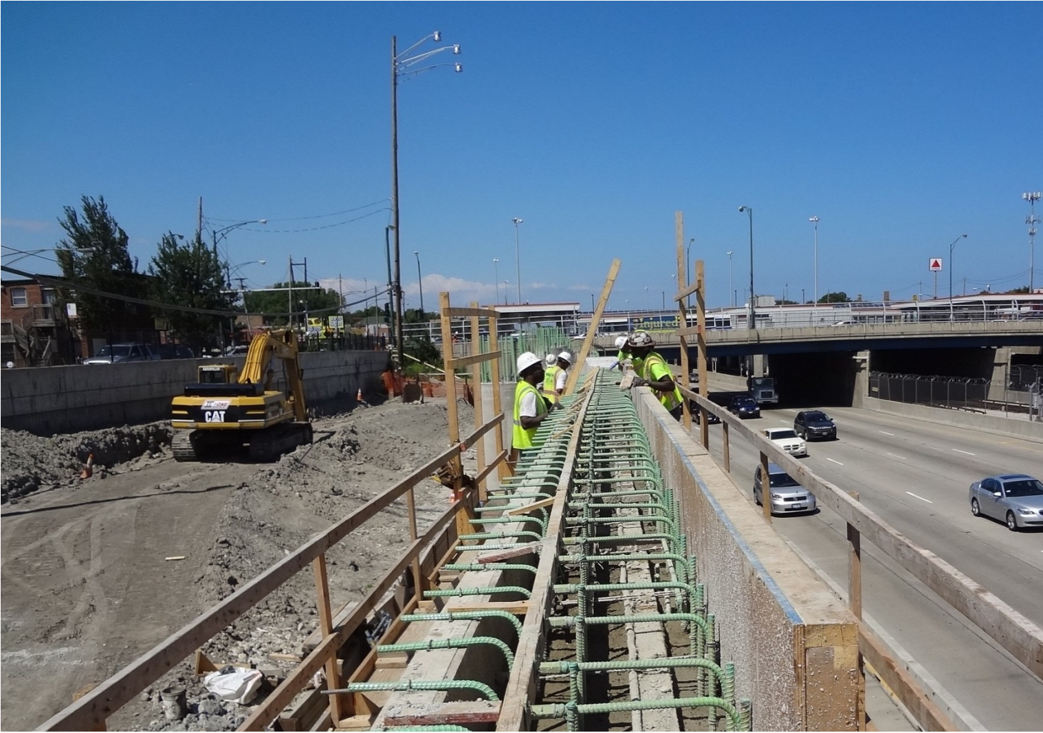
AP2: South Bus Bridge Back Wall Reinforcement (Wall 1)
