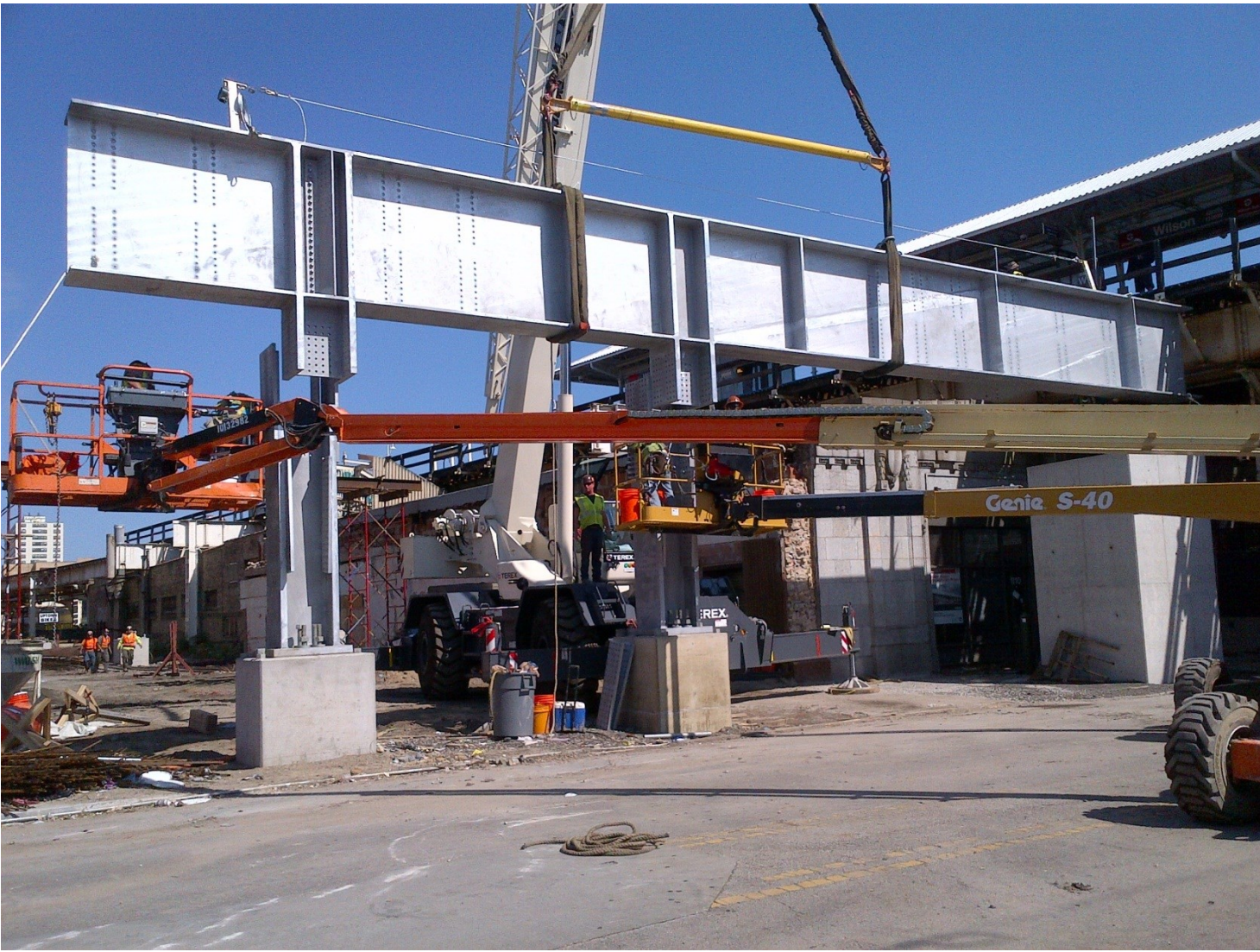
New structural steel bent installation
