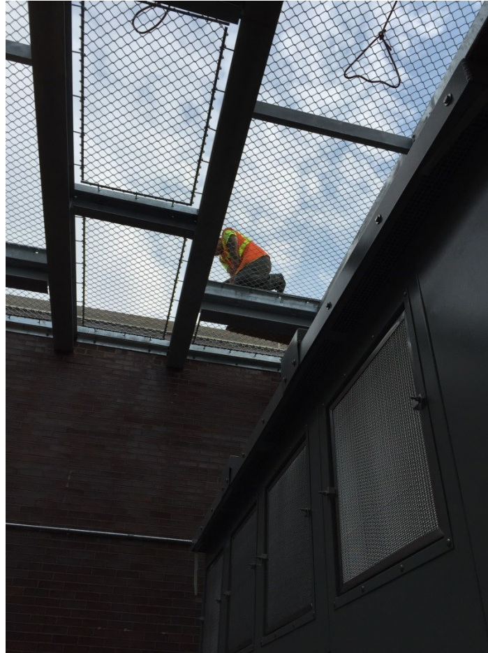
Kimball Substation: Installation of Courtyard Steel Mesh Panels
