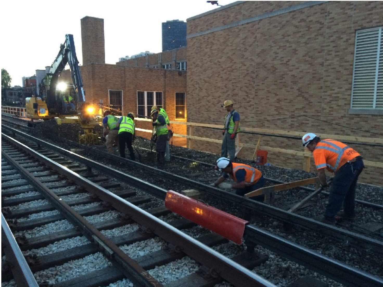
Track Four Tie Replacement
