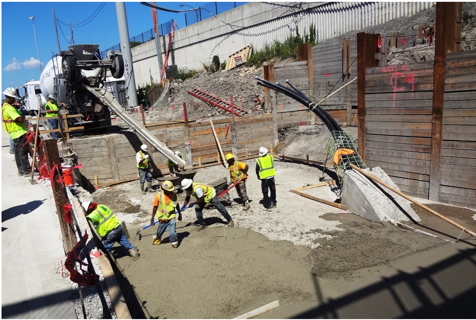
AP2: Backfill of East Side Jacking Pit (Wall 6)
