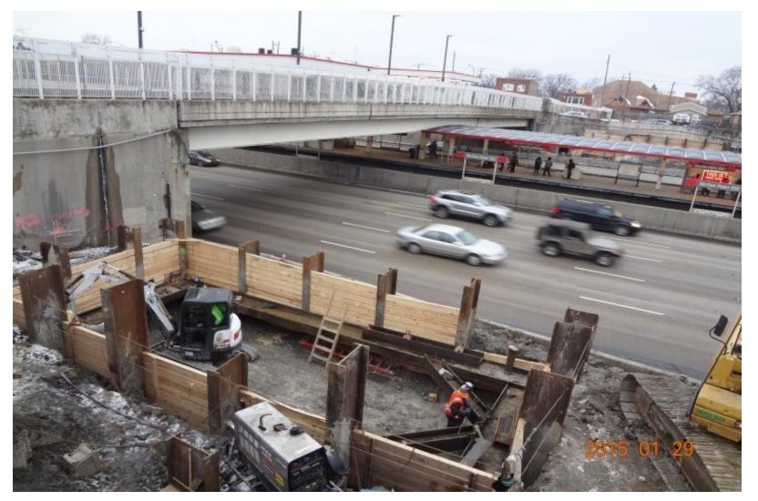
AP2: Northeast Quadrant (Wall 6) Earth Retention System for Jacking Pit for Fiber Optic and Electrical Ductbank under 95<sup>th</sup> Street
