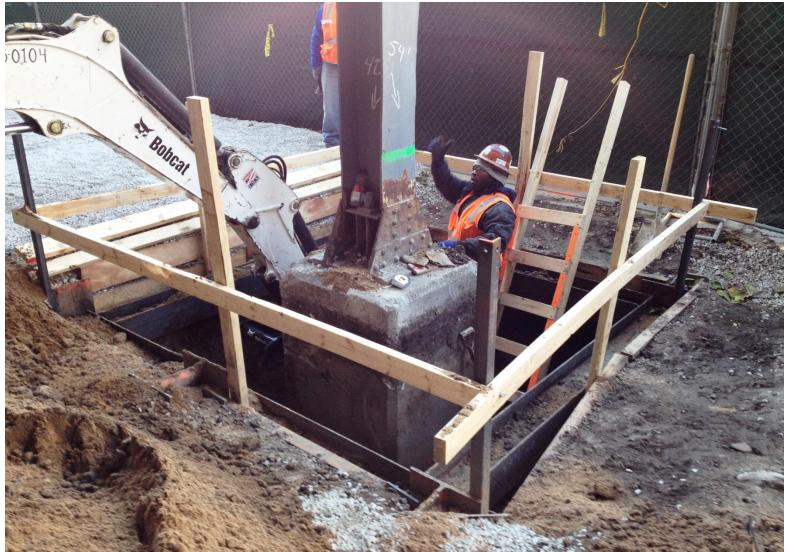
Armitage Substation: excavation around column base
