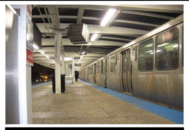
New Platform Canopy Light Fixture replacement. Platform Level view.
